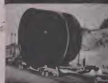
The outlet pipes were so big that they had to be manufactured on the spot, to avoid transportation difficulties
