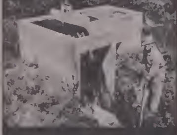
Cement-lined gravity ditches, waterfalls and steps led the water on down grades
