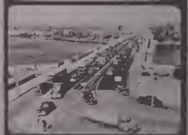
Many methods were tried before roads to withstand automobile speed were devised. Every road starts with clearing and leveling the road bed
