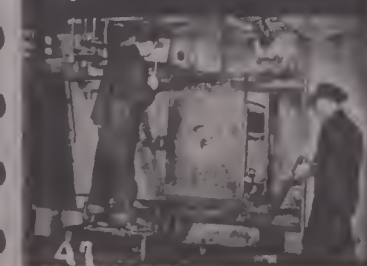
The roasting process is carefully watched - its main purpose is to burn off impurities and prepare the copper for smelting
