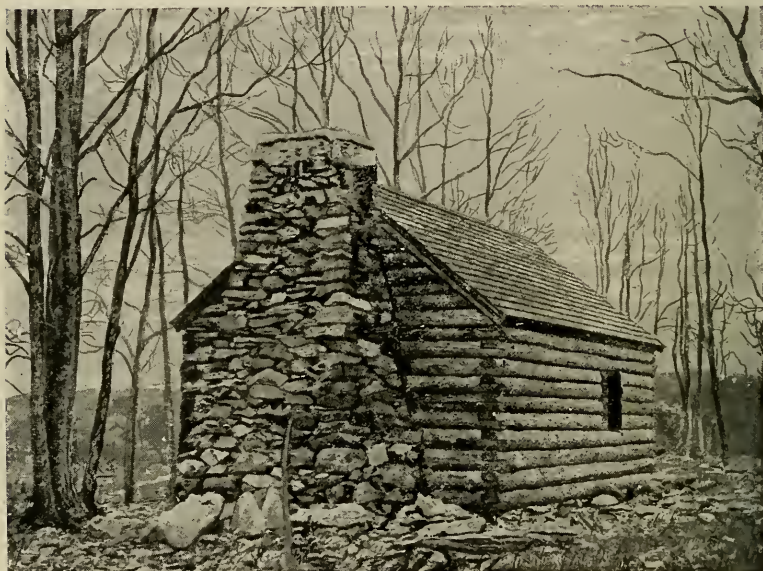
LOG CABIN, SITE OF GUARD HOUSE, PUTNAM CAMP
