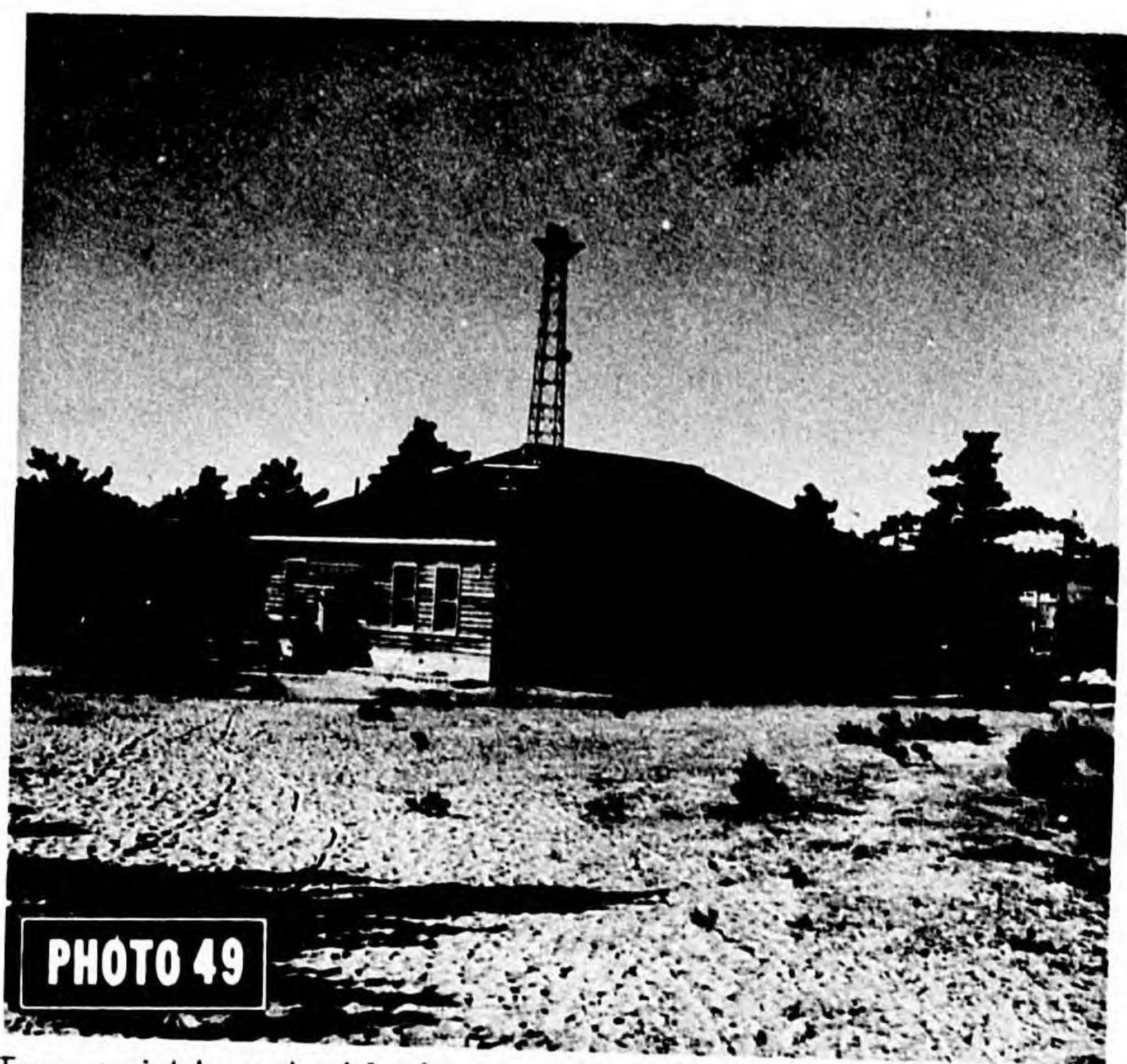
PHOTO 49 Transmitter building, near Fukuoka
