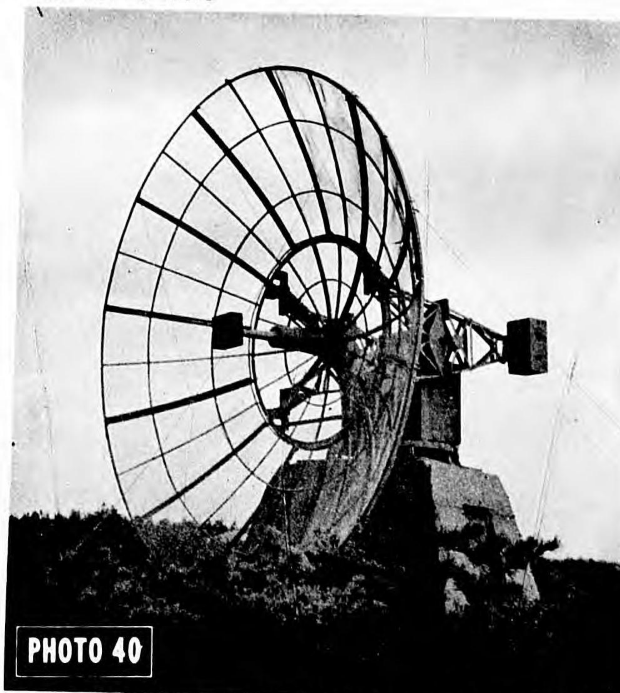
Army TACHI 24 copy of German Wurzburg, Tokyo area
