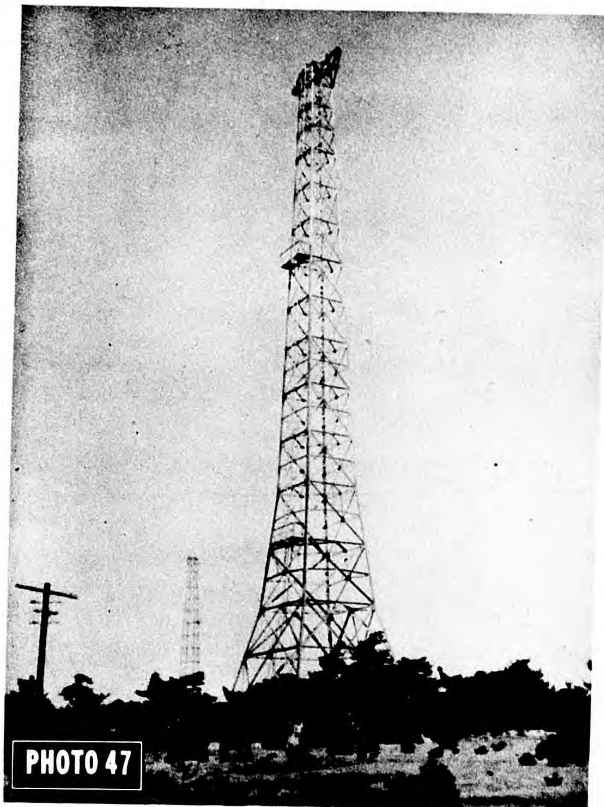
PHOTO 47 Lattice mast, near Fukuoka
