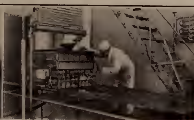
Dairy—Straining room, showing stairs to receiving room. Tubular cooler and bottler, with metal valves (no rubber), and operated entirely from the outside.
