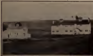
General view of the Milk House and large Cow Barn.
