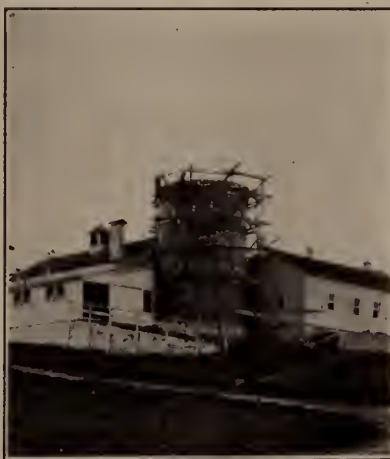
View of the small Cow Barns and Silo Tank, building.
