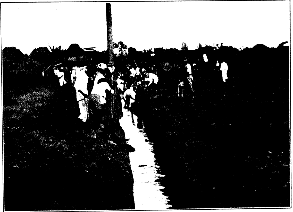
DRAINING SAN LAZARO ESTATE.
