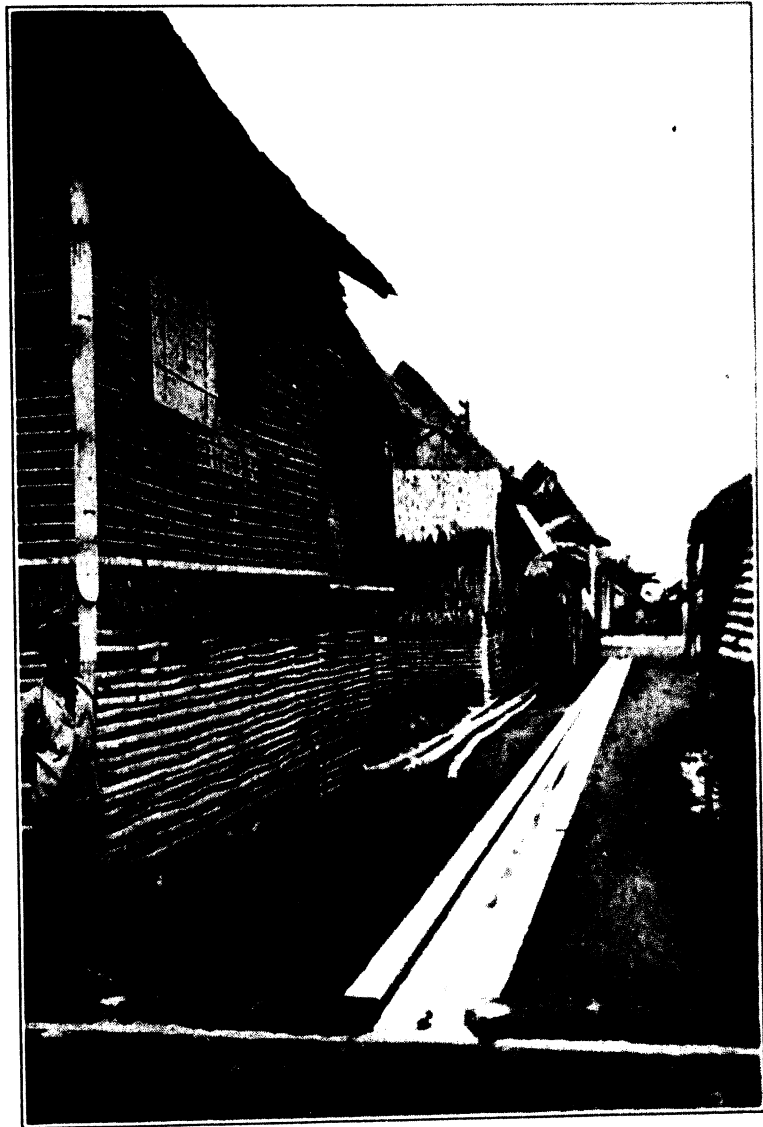
AN ALLEY IN SAN LAZARO ESTATE WITH NEW DRAINAGE SYSTEM.
