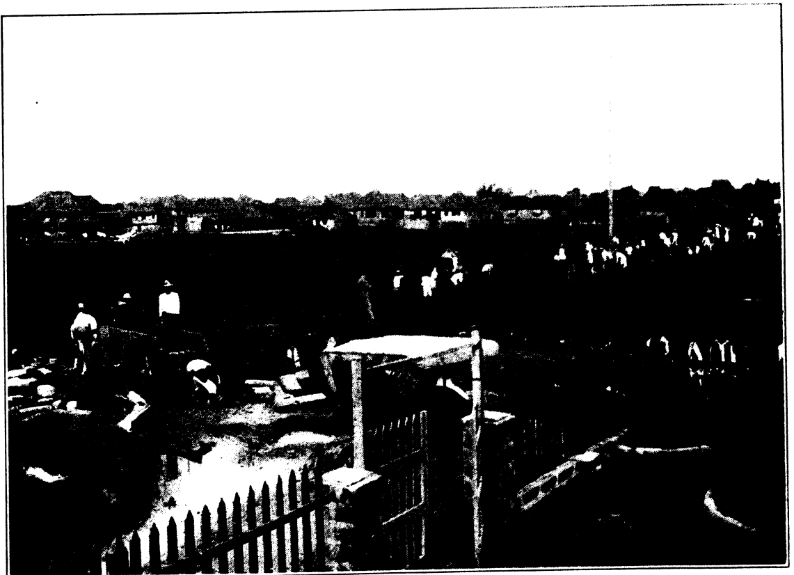
DRAINING SAN LAZARO ESTATE.
