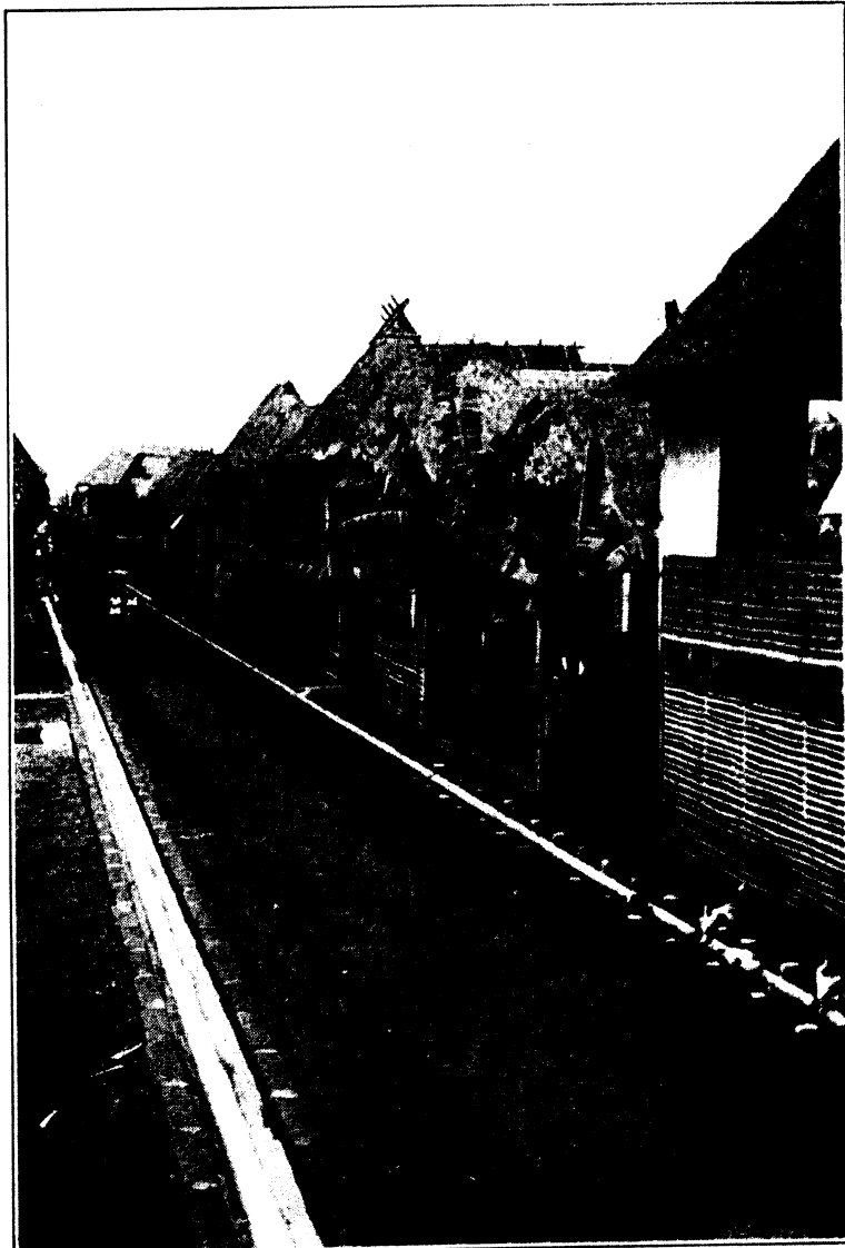
STREET IN SAN LAZARO ESTATE WITH NEW DRAINAGE SYSTEM.
