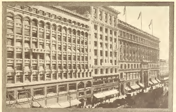
Down Town in Three Years!—Pacific, Commercial and Emporium Buildings.
