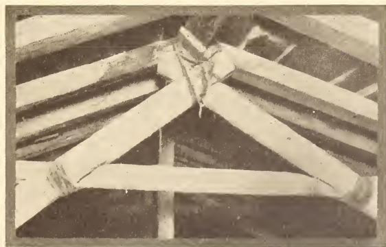
Beams in Roof Lashed Together With Rawhide Thongs.
