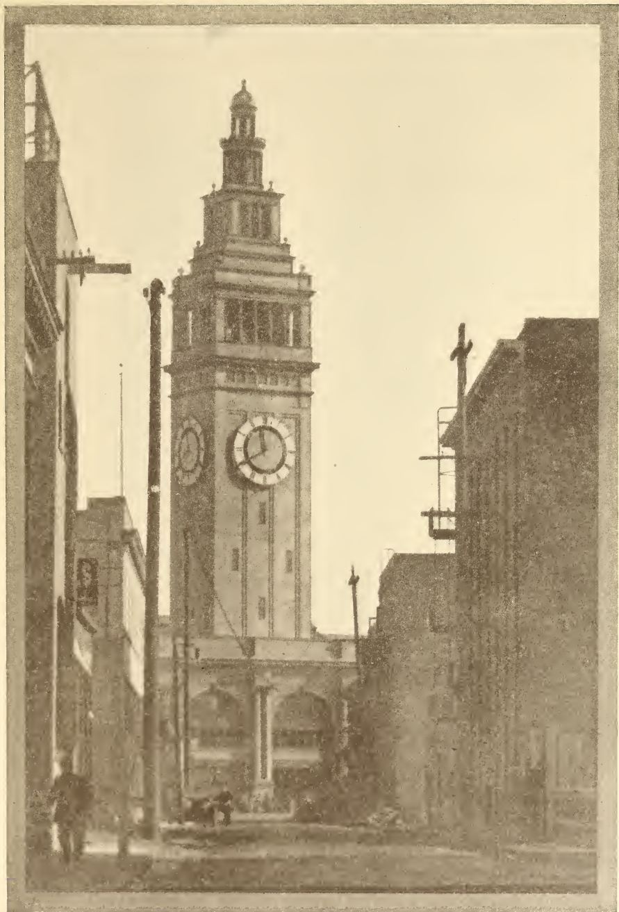
The Ferry Tower, Looking Down Commercial Street. Photograph by Louis J. Stellmann.
