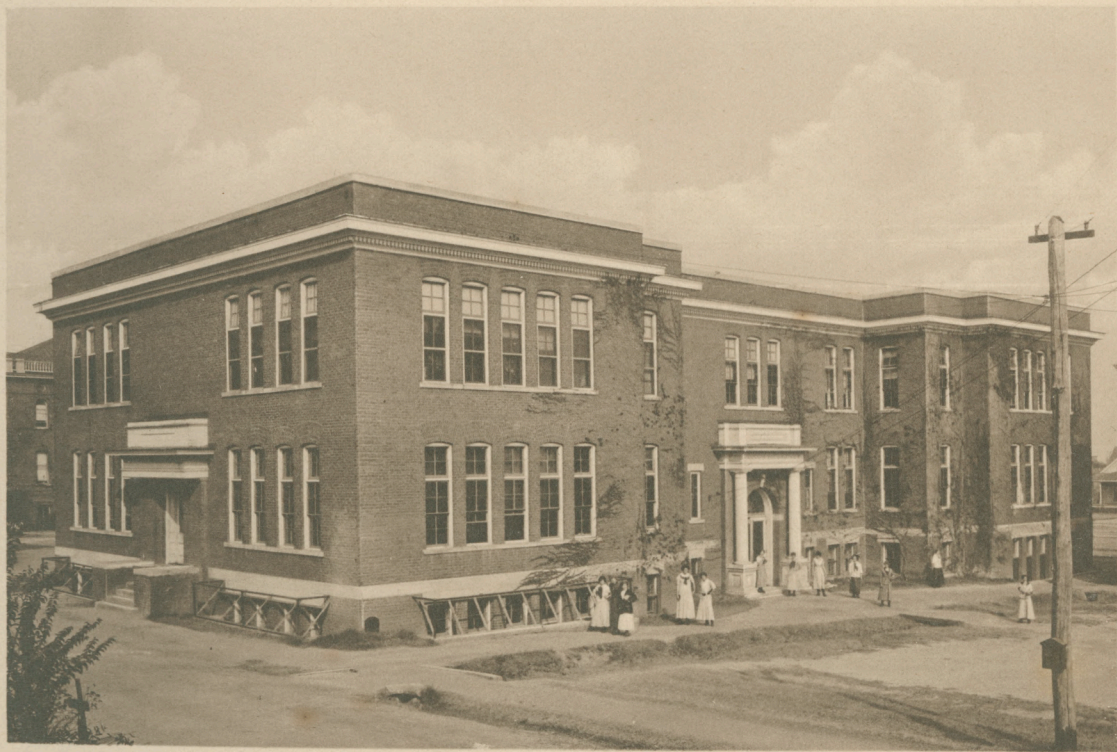
JAMES M. SMITH BUILDING.
