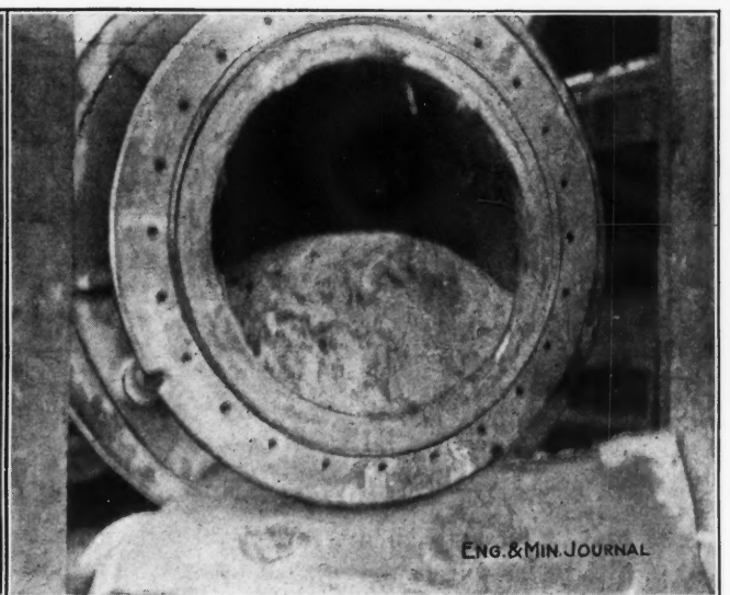
FIG. 9. CAKE OR LOAF READY TO DISCHARGE
