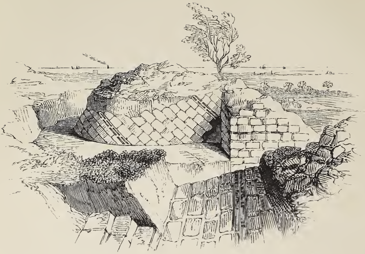
VIEW ON THE EASTERN SIDE.
