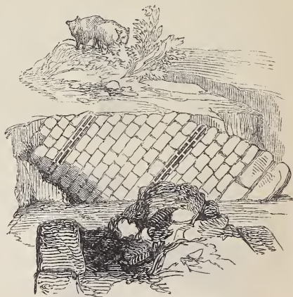
Postern entrance on the west.
