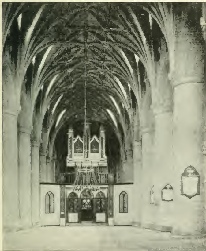
THE NAVE BEFORE RESTORATION.
