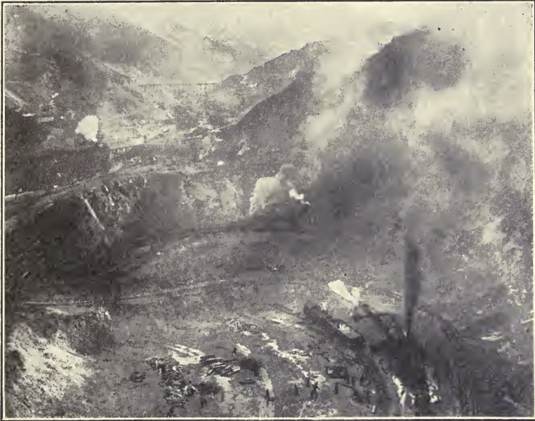
FIG. 11. — Steam shovels at work in pit of Utah Copper Company, Bingham, Utah.
