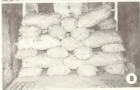
BN 23644, BN 23645 FIGURE 9. —Airflow pattern No. 5 for 100-pound burlap bags to provide air circulation channels; for use in either wide or narrow trailers. (A) First or header stack. (B) All subsequent stacks.
