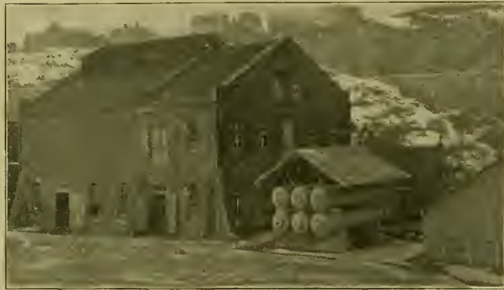
Fig. 1.—Exterior View of Plant.
