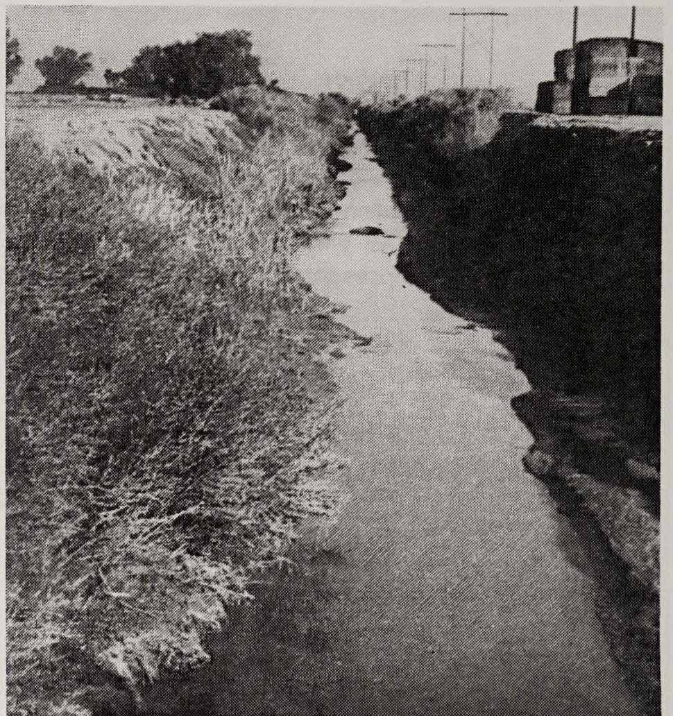
Photograph 2. Earthen drain along agricultural roads.
