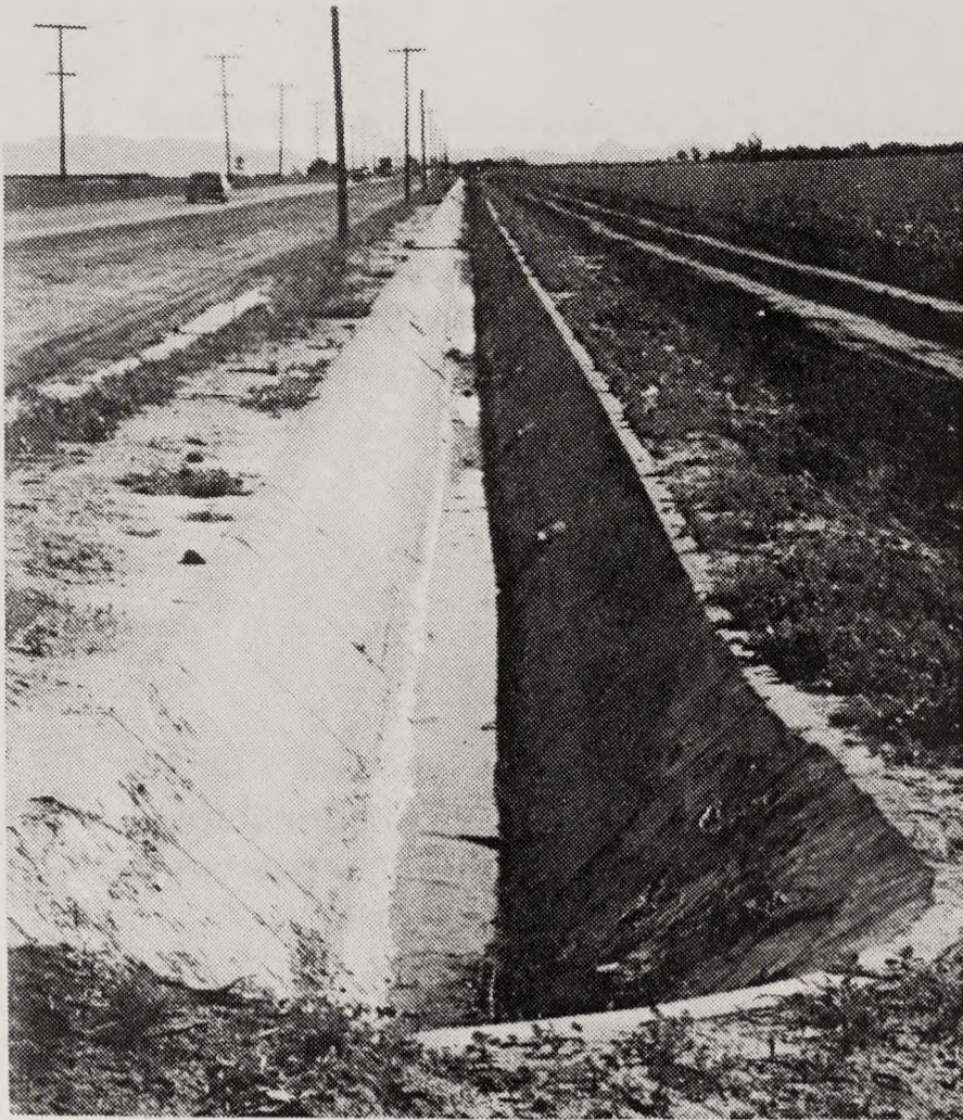
Photograph 1. Typical concrete-lined lateral along agricultural roads.
