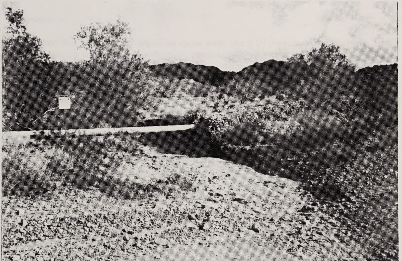
Photograph 2: Line 6000 exposed in desert wash along Gas Line Road.
