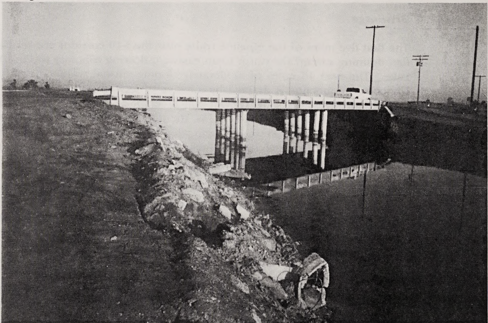
Photograph 3. Bowker Road crossing over Main Canal.
