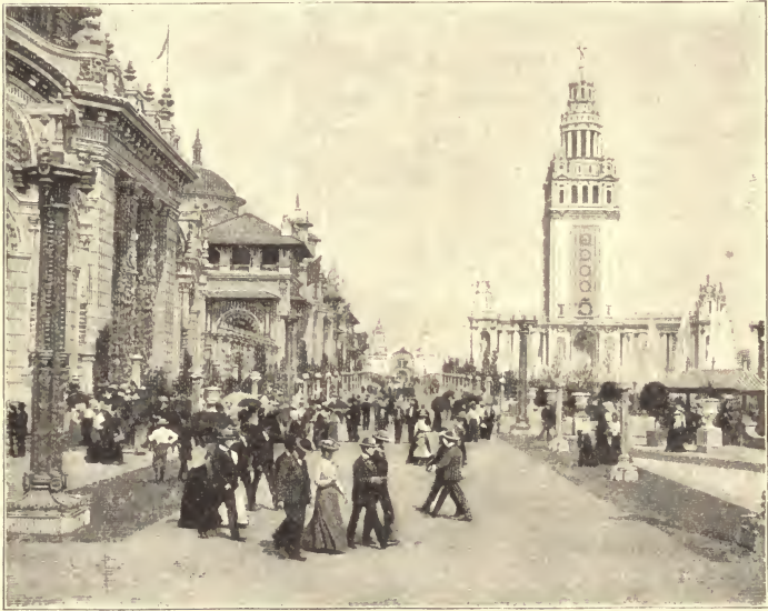
ELECTRIC TOWER, IN EXPOSITION AT BUFFALO, 1901.
