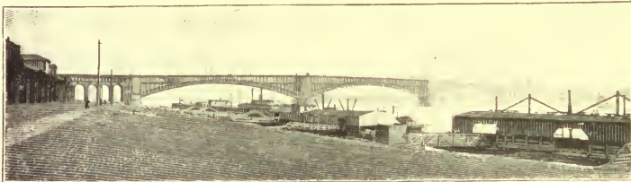
EADS STEEL BRIDGE, ST. LOUIS. (Spans, 520 feet.)
