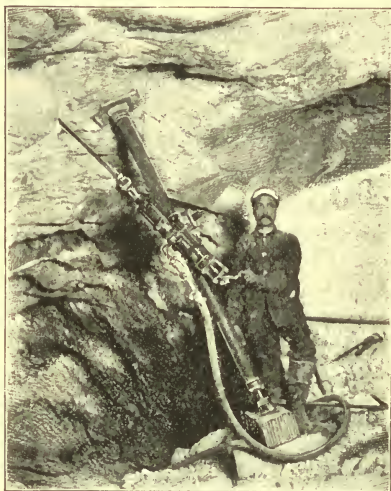
ROCK DRILL IN A CALIFORNIA GOLD MINE.
