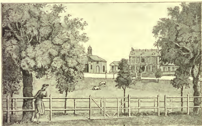
THE HANCOCK HOUSE IN 1789. From the Massachusetts Magazine .
