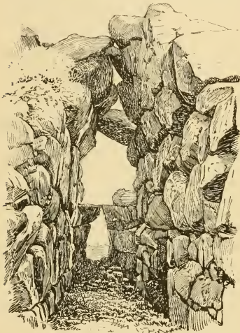
WALL OF TIRYNS.
