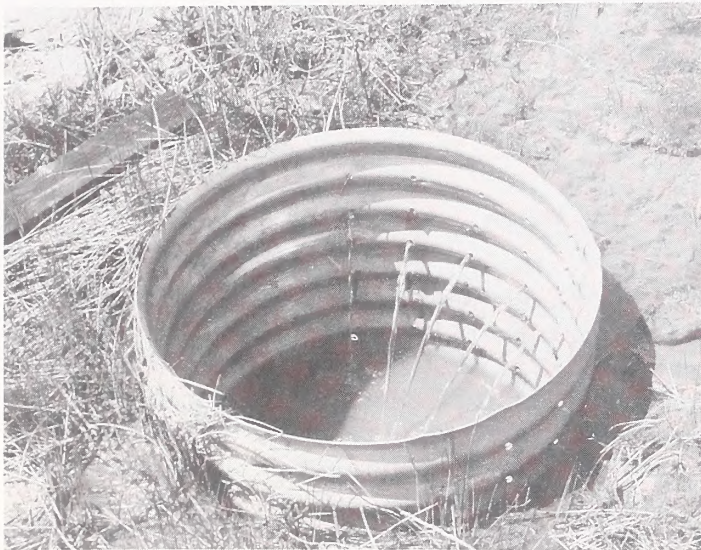
A lowcost storage tank collecting snowmelt.
