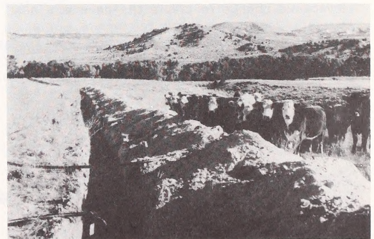
Water pipeline under construction.
