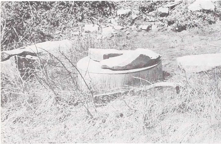
A water storage tank with a well-anchored roof (to minimize evaporation).
