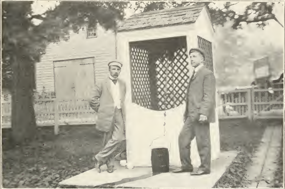
At the old homestead of Captain Abraham Shimer, in the Valley of the Minisink, now Montague, N. Y. This well was dug, as far as we could learn by the Captain, when he built his house, 1750, the first two-story dwelling in the township.
