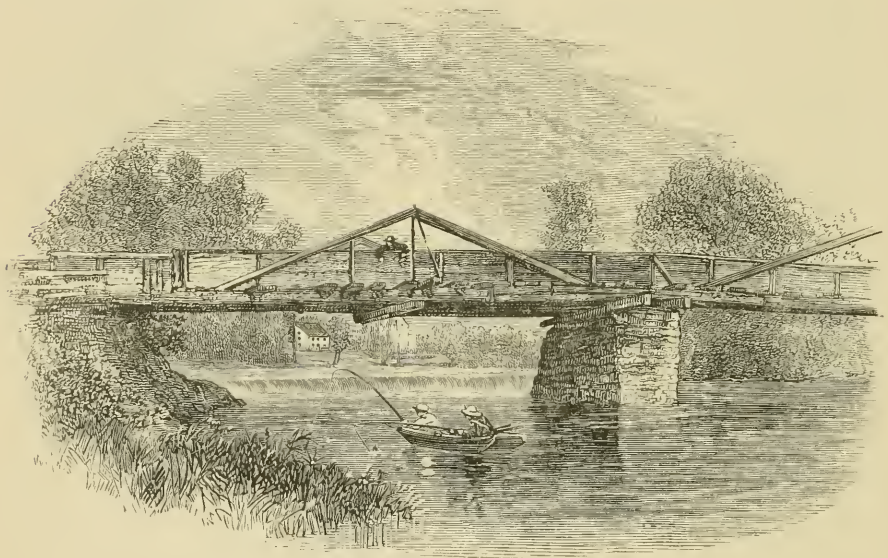
RUSTIC BRIDGE, NORWICH.
