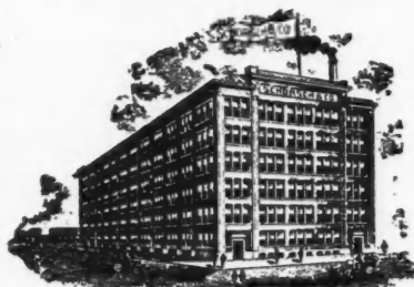
FACTORY 132 ND TO 133 RD ST. & BROOK AVE
