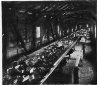
Belt Conveyor Handling Coal
