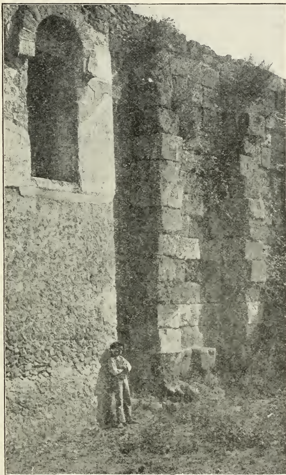
Fig. 109.—View of the city wall, inside, where the embankment has been removed. The door in the tower at the left marks the height of the embankment.
