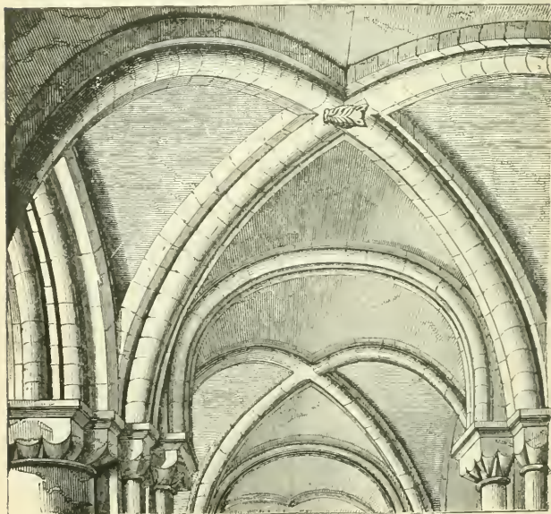
62. Peterborough Cathedral, A.D. 1117—1143. Norman Vault with arch-ribs and groin-ribs.
