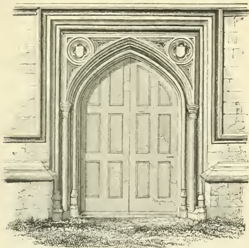
155. Fotheringhay, Northamptonshire, A.D. 1440.
