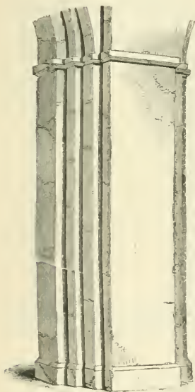
40. St. Alban's Abbey, A.D. 1030. Early Norman Pier, recessed and square-edged.
