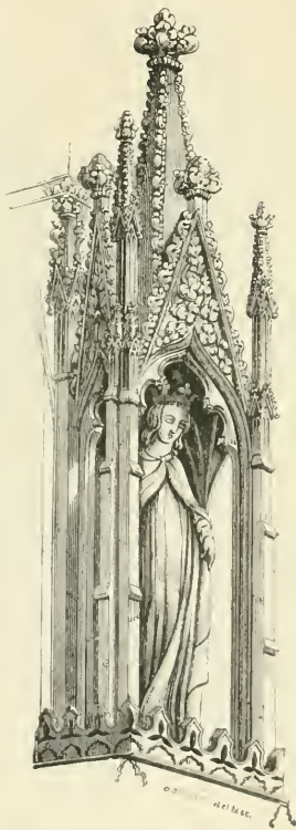
139. Open Niche, with Canopy and Pinnacles, and Figure of Queen Eleanor, from her Monumental Cross at Northampton, A.D. 1294.
