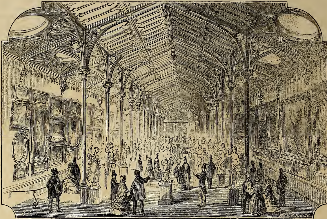
INTERIOR VIEW OF THE NEW GALLERY.
