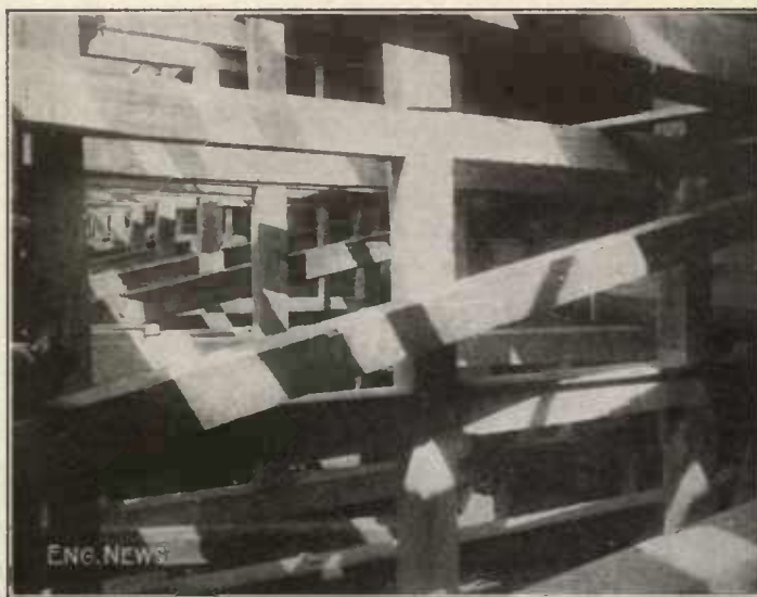
FIG. 35. TIMBERING IN EARTH EXCAVATION AT LEFT AND ROAD EXCAVATION AT RIGHT, ON LEXINGTON AVE.
