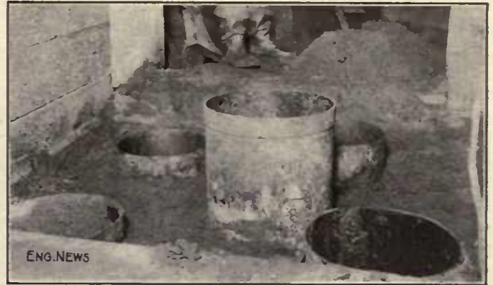
FIG. 65. HOLLOW PILES FOR FOOTING OF ELEVATED-RAILWAY COLUMNS
