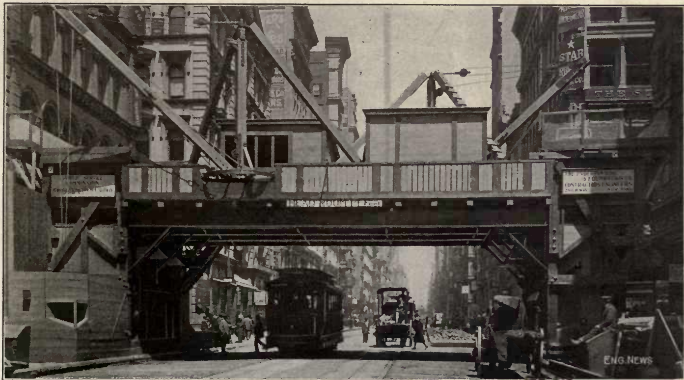
FIG. 47. BRIDGE AND DERRICKS AT GRAND ST. AND BROADWAY
