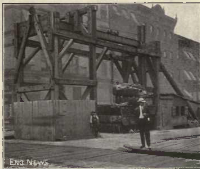
FIG. 44. GANTRY HOIST FOR SKIPS AT 121ST ST. AND LEXINGTON AVE.
