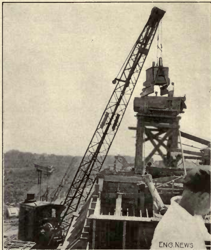
FIG. 89. LIFTING CONCRETE BUCKETS INTO PLACE, QUEENS BOULEVARD VIADUCT
