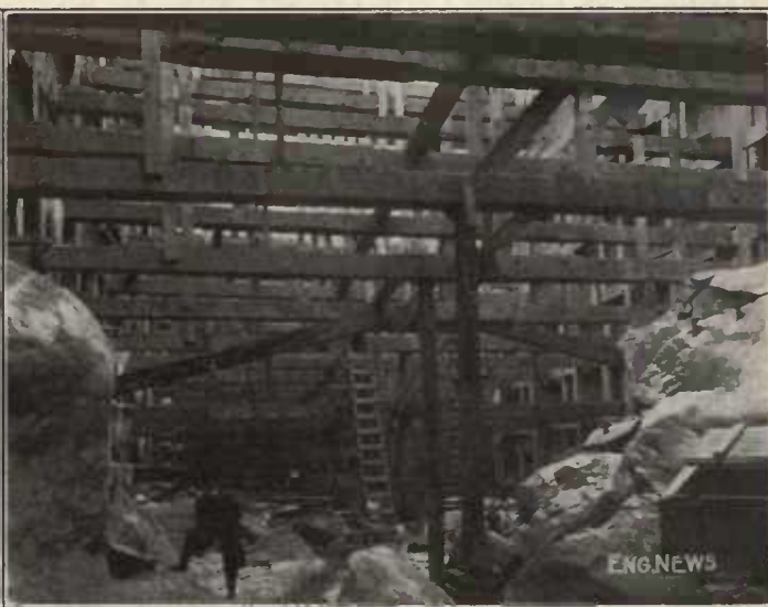
FIG. 35. TIMBERING IN EARTH EXCAVATION AT LEFT AND ROAD EXCAVATION AT RIGHT, ON LEXINGTON AVE.
