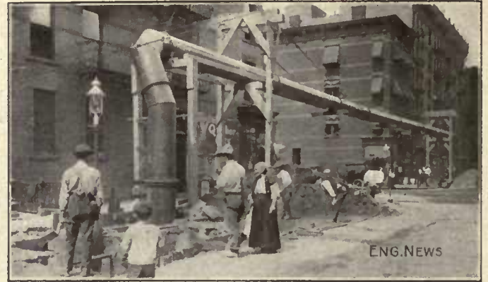
FIG. 27. OVERHEAD GAS MAIN AT LEXINGTON AVE. AND 112TH ST.
