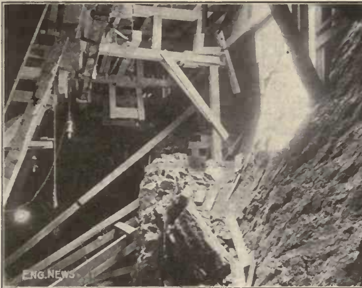
FIG. 51. A ROCK SLIDE, LEXINGTON AVE. SUBWAY
