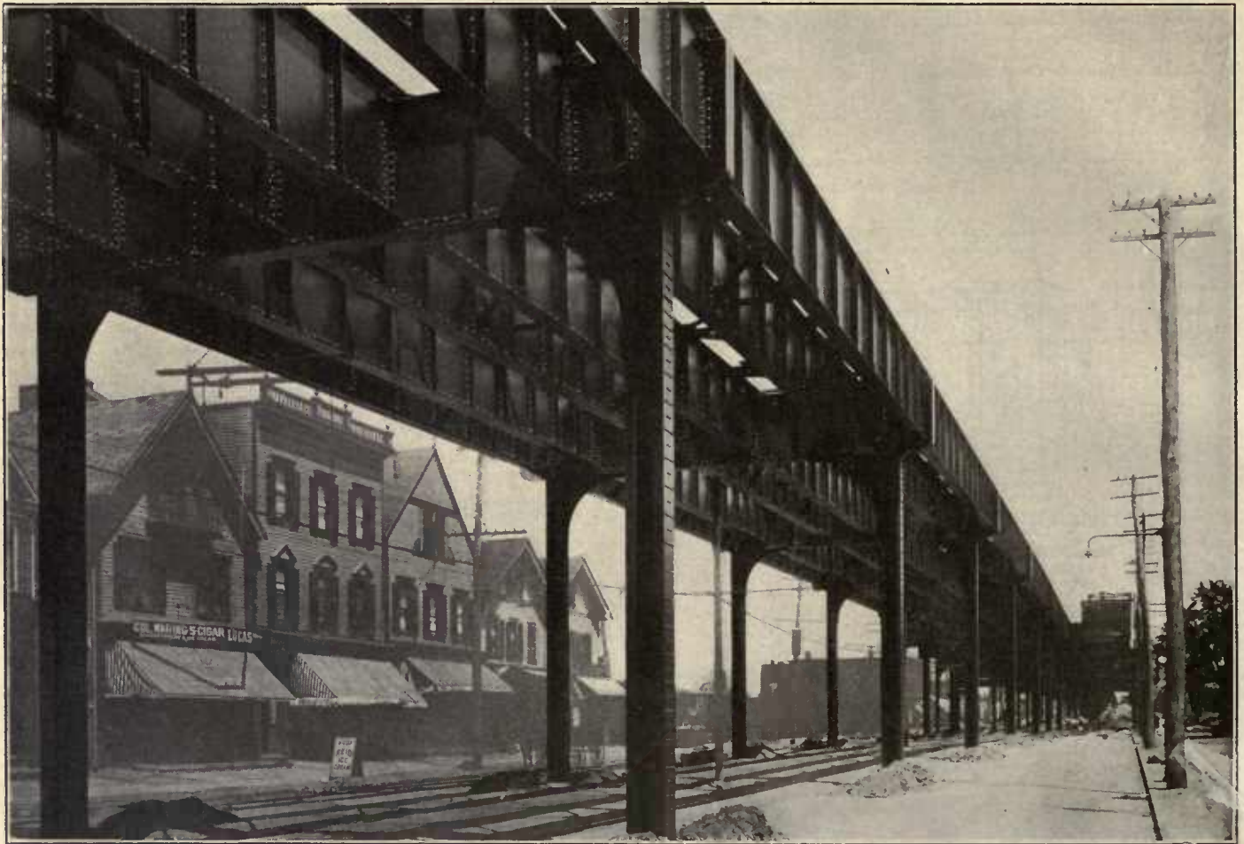
FIG. 94. NEW ELEVATED STRUCTURE WITH COLUMNS IN STREET (WHITE PLAINS ROAD, BRONX BOROUGH)
