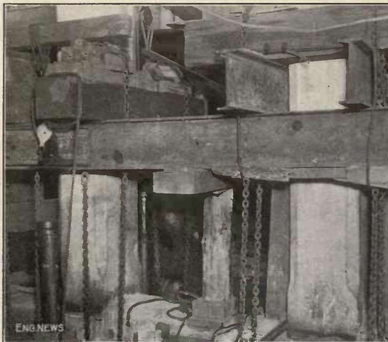
FIG. 57. UNDERPINNING WITH NEEDLES BUILDING AT 459 BROADWAY
