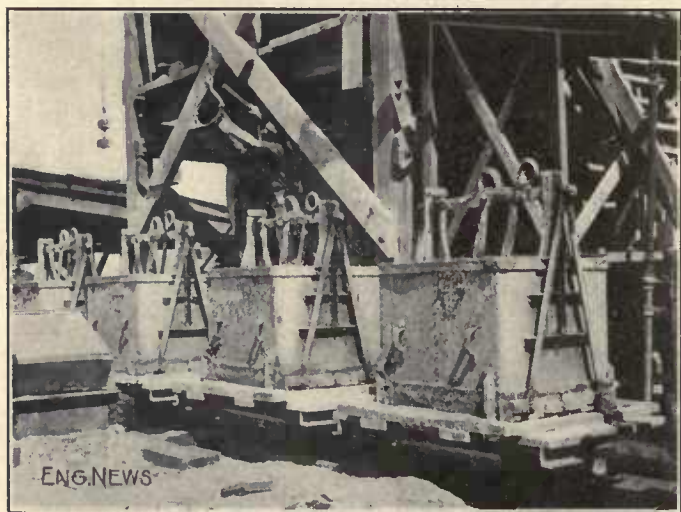
FIG. 88. CONCRETE BUCKETS ABOUT TO BE LOADED
