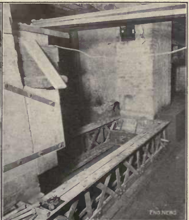
FIG. 58. UNDERPINNING WITH A LATTICED GIRDER
