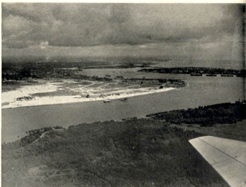
APAPA RECLAMATION SCHEME, LAGOS
