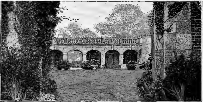
Bulwick, covered way.
