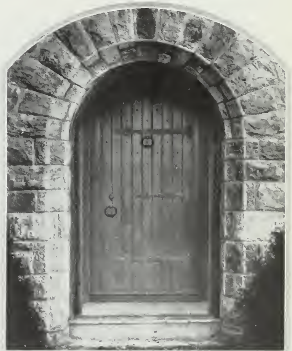
Front Entrance Door. Each stone whether for trim work or for the walls was chosen for its perfection in color and texture.
