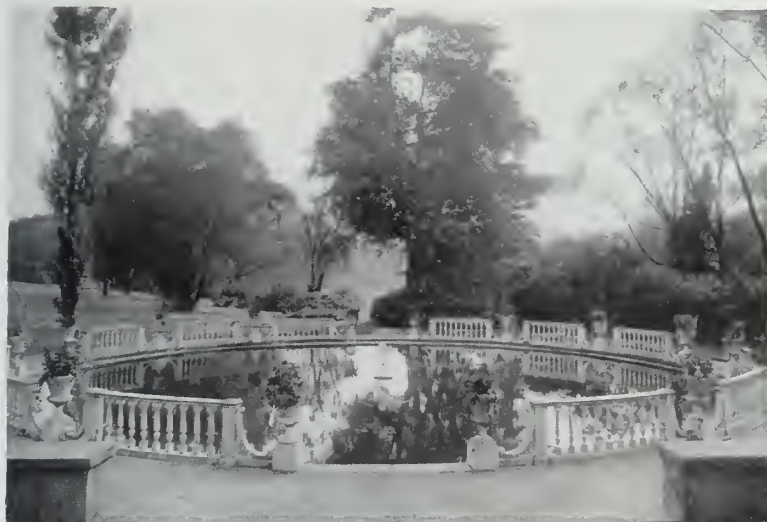
LOUIS S. ADAMS, ARCHITECT
