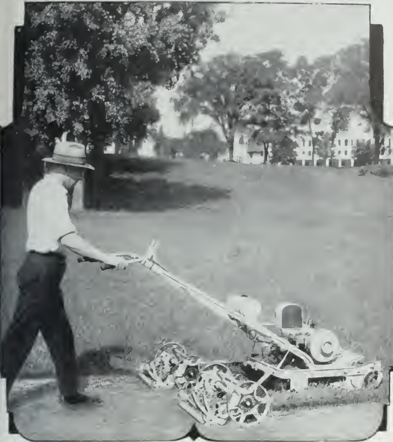
Above: Coldwell "L-Twin" motor lawn mower and roller. Mows and rolls simultaneously 4 to 6 acres a day on one gallon of Gasoline. Gang units more than double its capacity.
