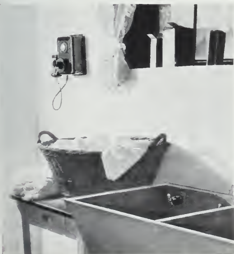
In the laundry, a handy telephone saves many a climb up and down the basement stairs.
