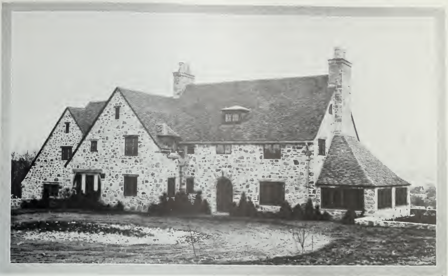
Norman antique tile roof. Solid oak beams over all outside windows. Connecticut field stone walls. A house of distinction from footings to ridgepole.
