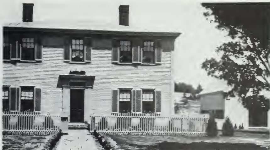
The plain simple lines of the old "starch box" houses were an indication of the airy, comfortable rooms behind their rather severe fronts. Remodeling of these old houses presents no particular difficulties.
