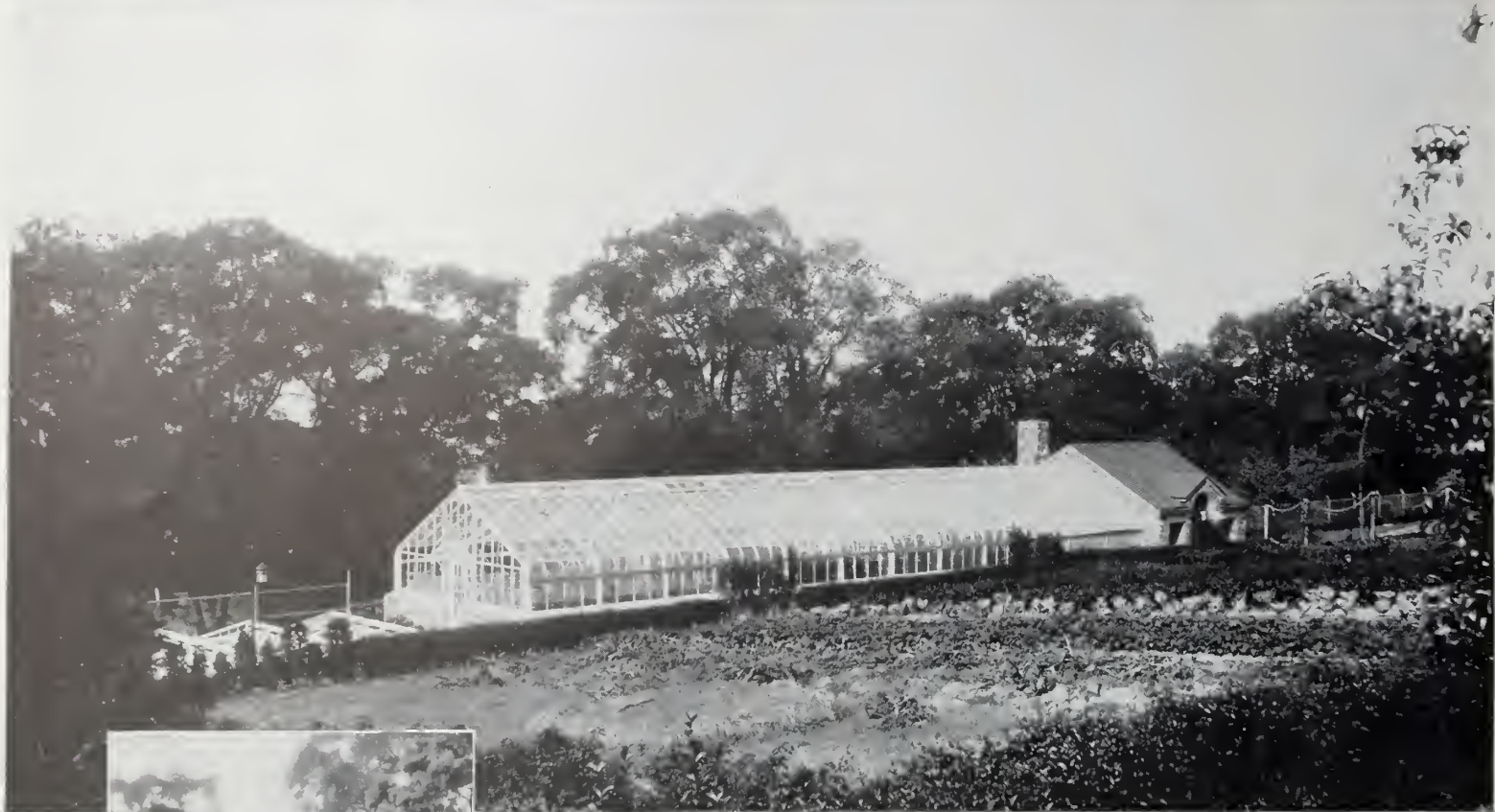
The glass garden portion is 25 feet wide and 100 long, divided into four separate compartments
