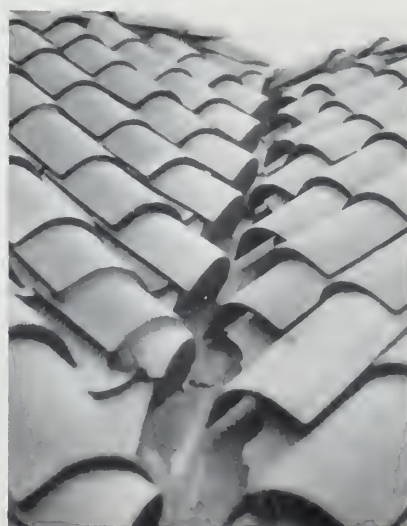
A poorly laid tile roof. The flashing was too narrow and not carefully turned, and the tile ends were left open. Tile is an excellent roofing material when properly installed
