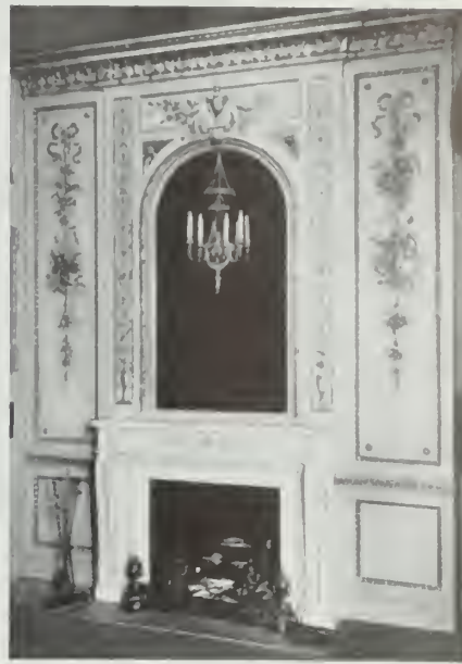
The rich and delicate mantel decoration shown above is secured by applying "Compo"
