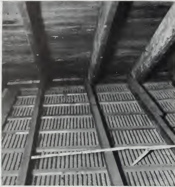
Improper construction of roof framing. Too light timbers were used to support the ceiling and tie the rafters together to strengthen the roof, and these were spaced too far apart. In this house the ceilings of the bedrooms cracked and partially fell off
