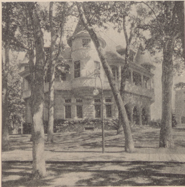
MAINE BUILDING, POLAND SPRING
