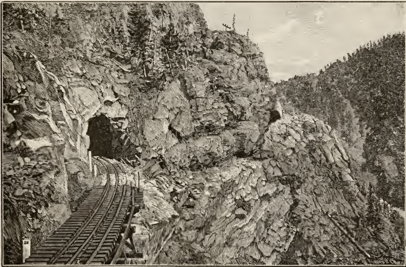
WEST END OF THE TOLTEC TUNNEL.
