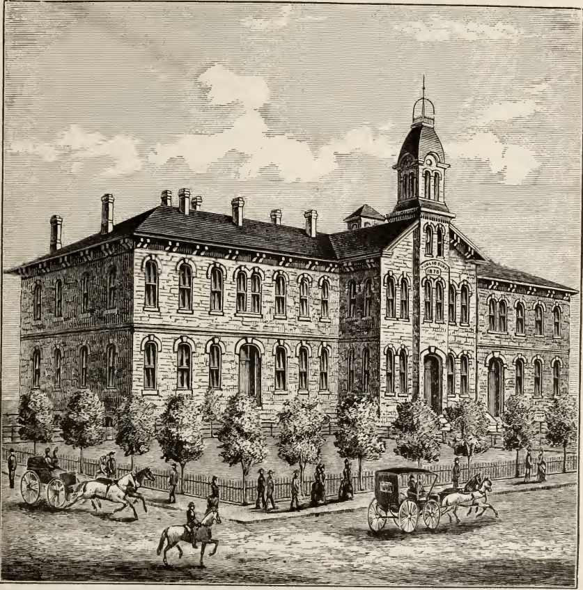
CENTRAL SCHOOL BUILDING.
