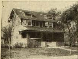
A No. 3015 IDEAL Boiler and 175 ft. of 38-in. AMERICAN Radiators, costing the owner $125, were used to Steam heat this cottage.
