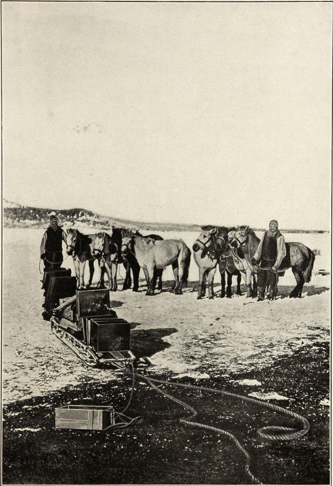
THE MANCHURIAN PONIES USED BY SHACKLETON INSTEAD OF DOGS FOR THE SOUTHERN SLEDGE TRIP. THEY PROVED A REMARKABLE SUCCESS. THEY WERE WELL FED UNTIL THE FOOD BEGAN TO GIVE OUT, WHEN THEY WERE KILLED, AND THEIR FLESH WAS EATEN OR DEPOSITED IN DEPOTS
