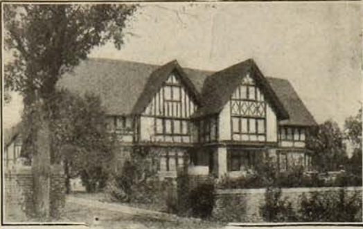
Stained with Cabot's Shingle Stains Robert C. Spencer, Jr., Architect, Chicago
