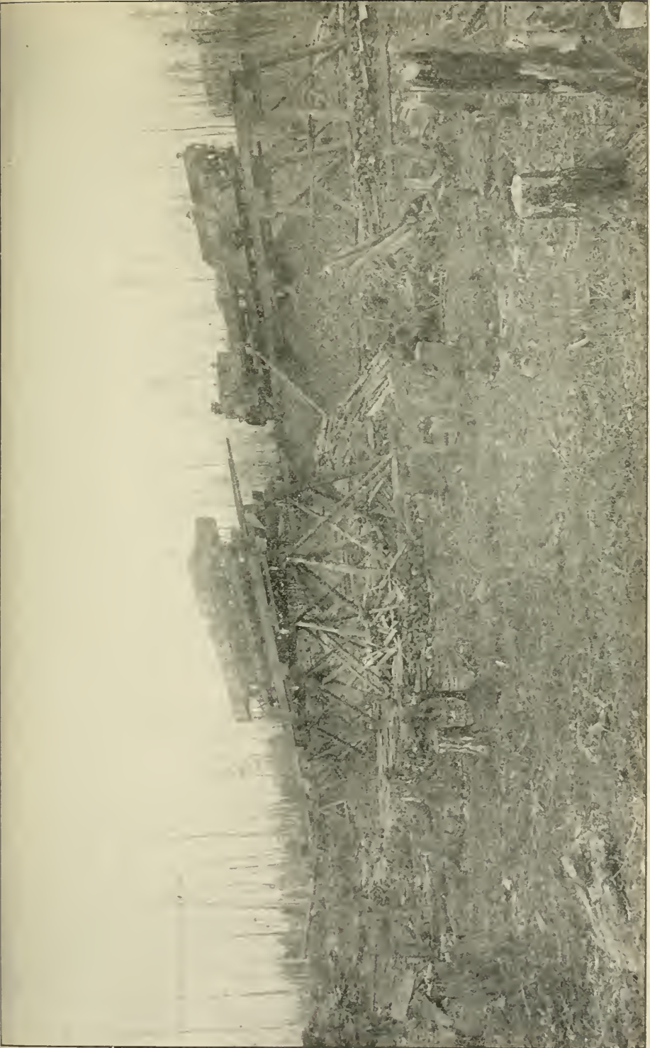
Box-heaps at Gertrude nickel mine, showing method of constructing heaps.
