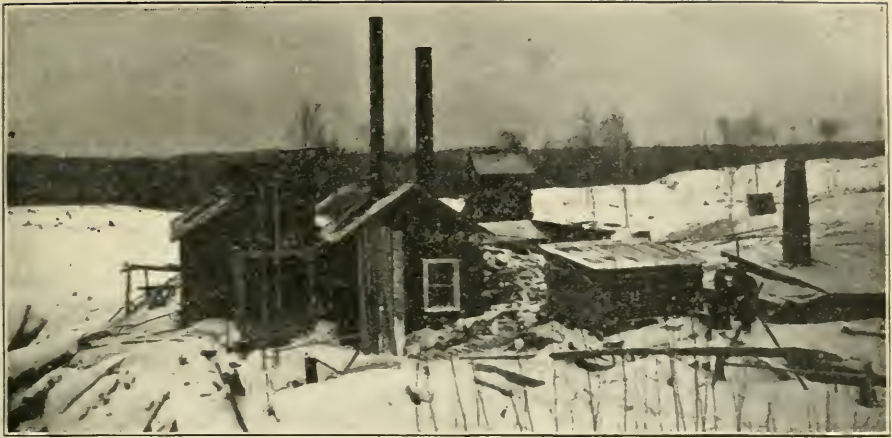
Grace gold mine from north, showing shaft and power houses.
