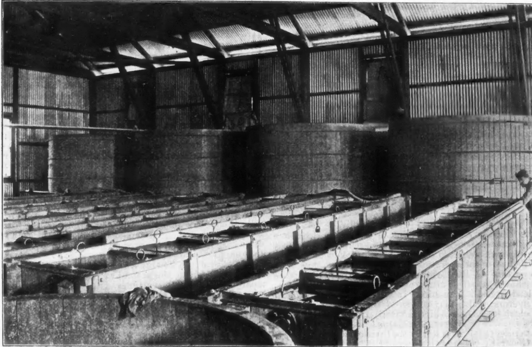
EXTRACT HOUSE, NEW PRIMROSE MINE, TRANSVAAL.
