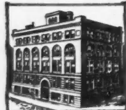
Machinery Hall, Armour Inst.
