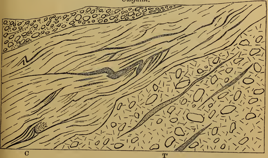
Fig. 4.—Section in the Settle and Carlisle Railway-cutting at Culgaith.
