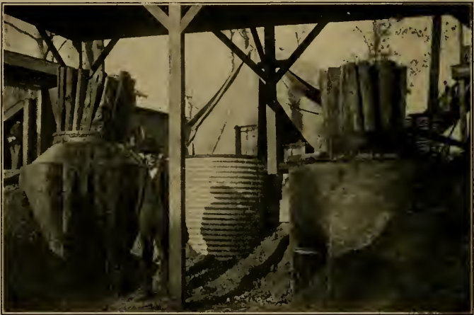
FIG. 54.—A United States Forest Service plant for the preservative treatment of fence posts.
