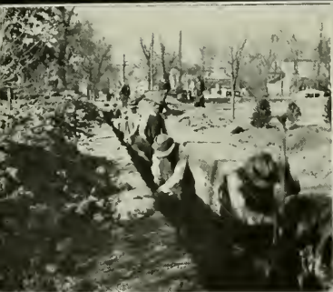
DIGGING UP THE WALKS
