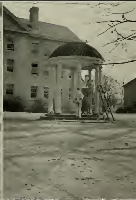
REPAIRS FOR THE OLD WELL
