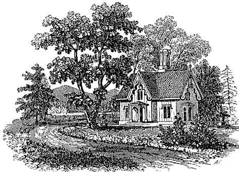
[Fig. 60. The Gardener's House, Blithewood.]
