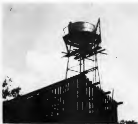
PUMPING STATION AND WATER TANK FOR IRRIGATION PUR- POSES
