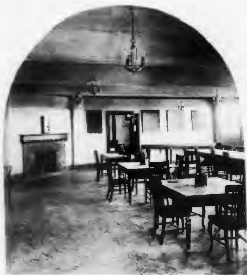
Courtesy of The Foundation Company
