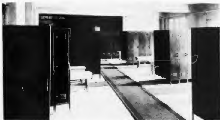
Courtesy of The Foundation Company
