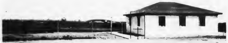
Courtesy of The Foundation Company
