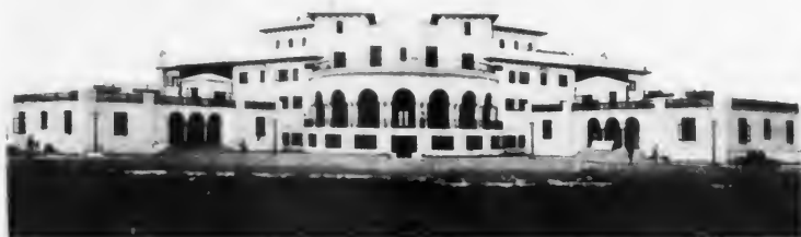
Courtesy of The Foundation Company
