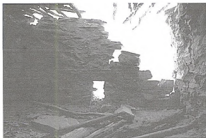
Figure 2. Paired views taken from the inside of a structure on an ancestral Pueblo site in Glen Canyon National Recreation Area. In 1978, most of the front wall was intact and the foundation was solid (View A, left). By 1997, the front wall had been completely destroyed (View B, right).
