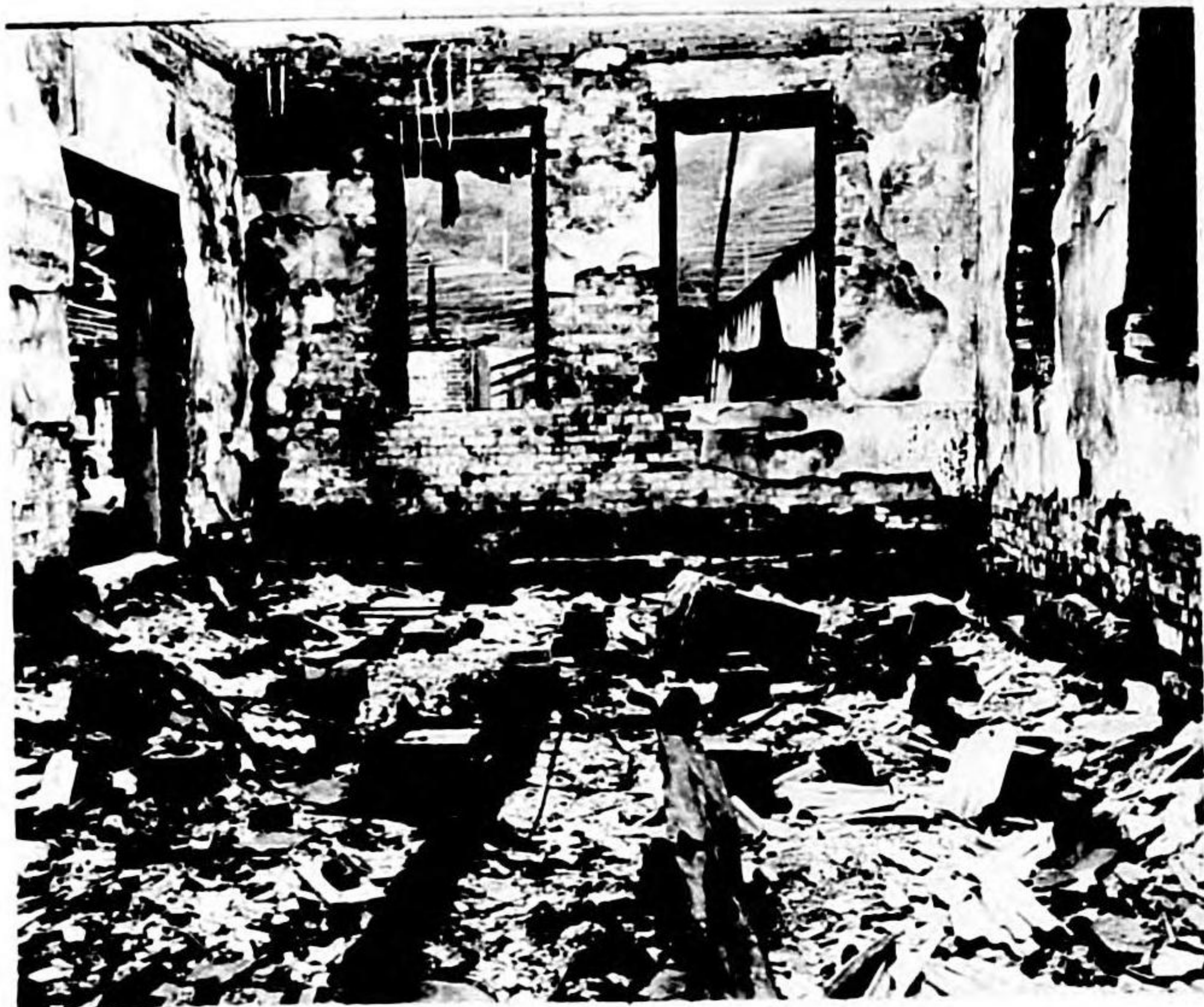
Photo 194. Nagasaki. Load-bearing brick-wall structure, 6,400 feet from GZ. Roof and contents destroyed by fire.
