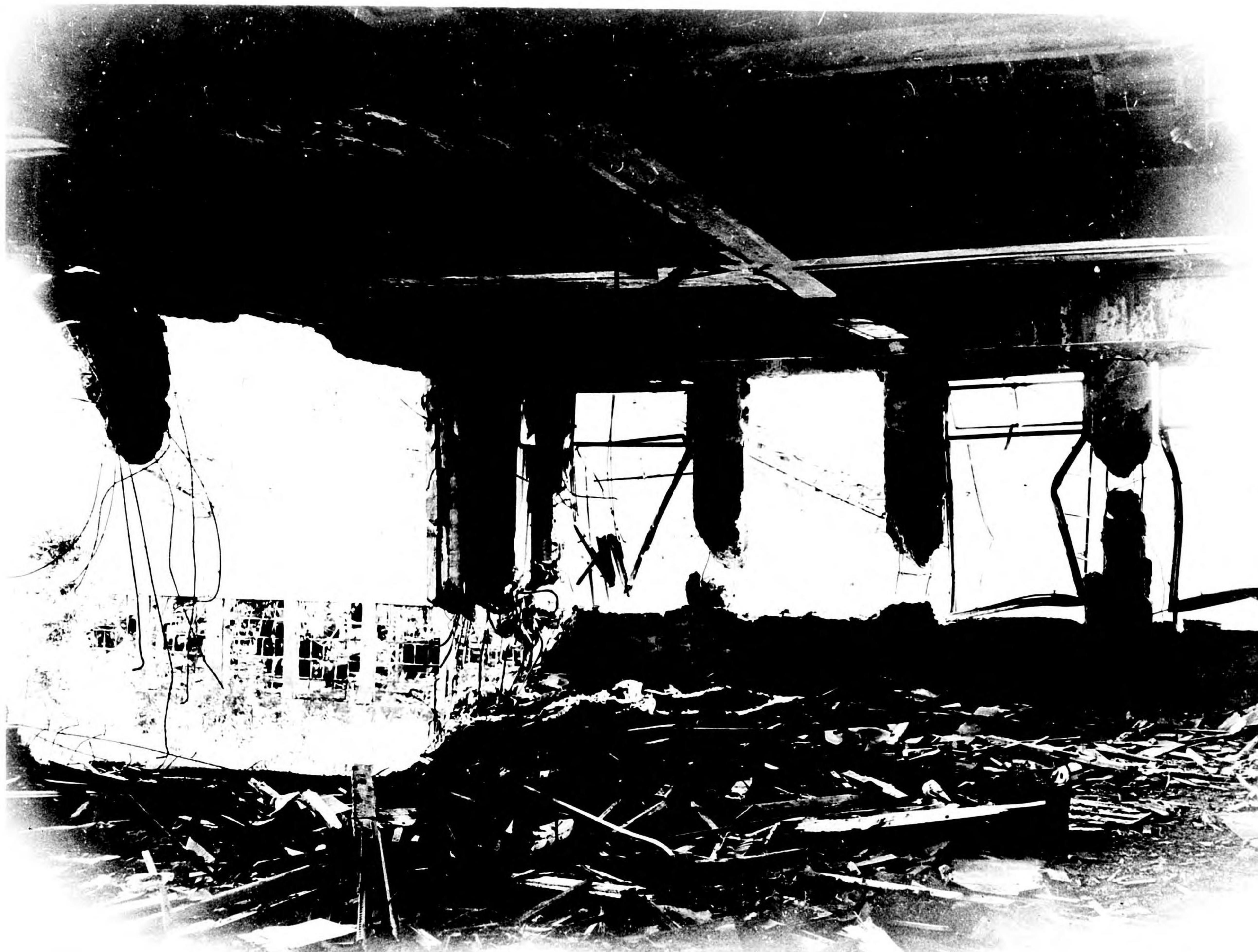
Photo 205. Interior columns of three-bay-wide building severed, also a corner column and sections between windows, but third-floor-and-roof section cantilevered out from undamaged part.
