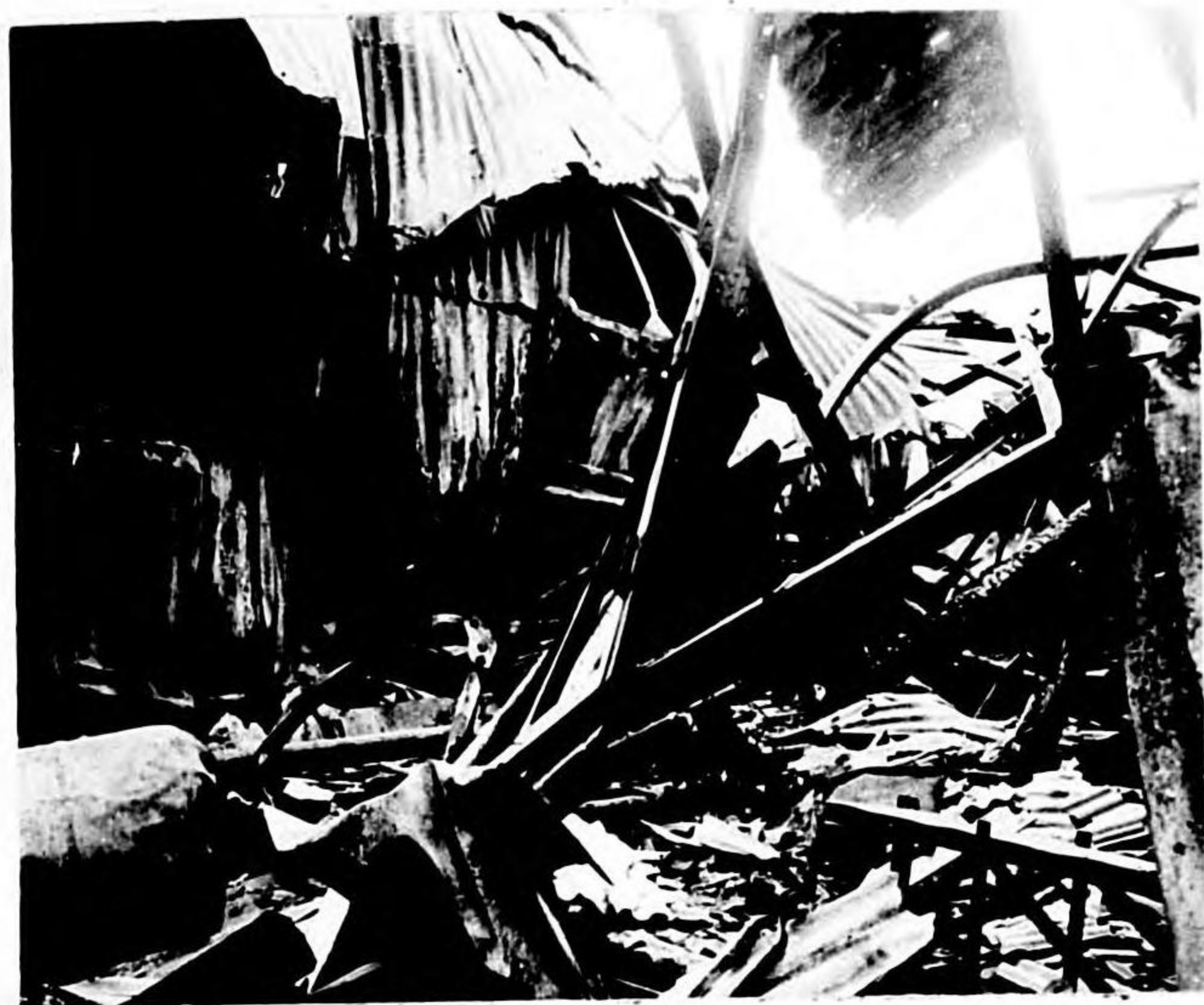
Photo 193. Nagasaki. Steel-frame building 6,300 feet from GZ. Damage by blast and fire. Effect of intense heat on steel trusses.
