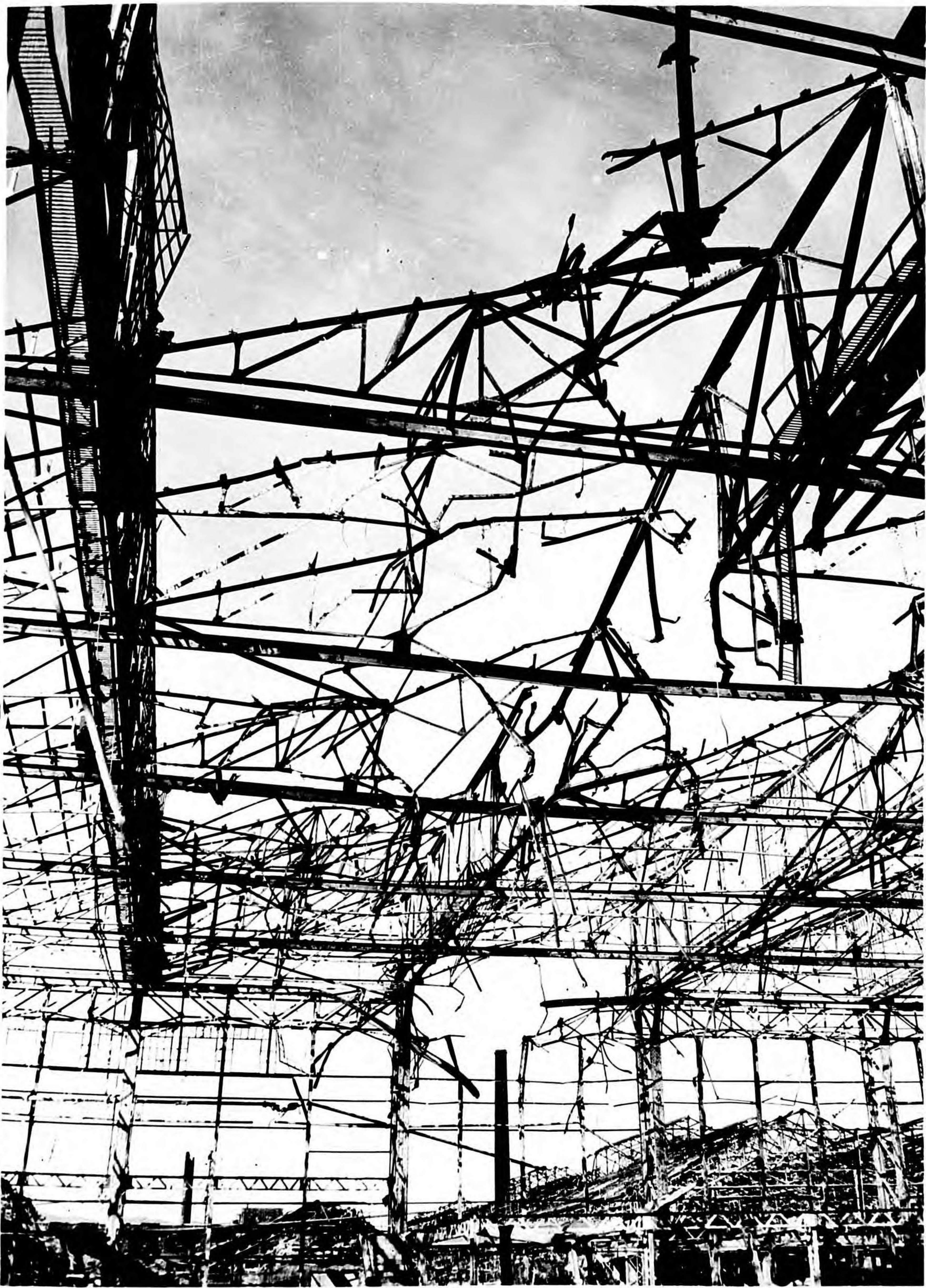
Photo 195. Gnawing action of four 500-pound bombs.
