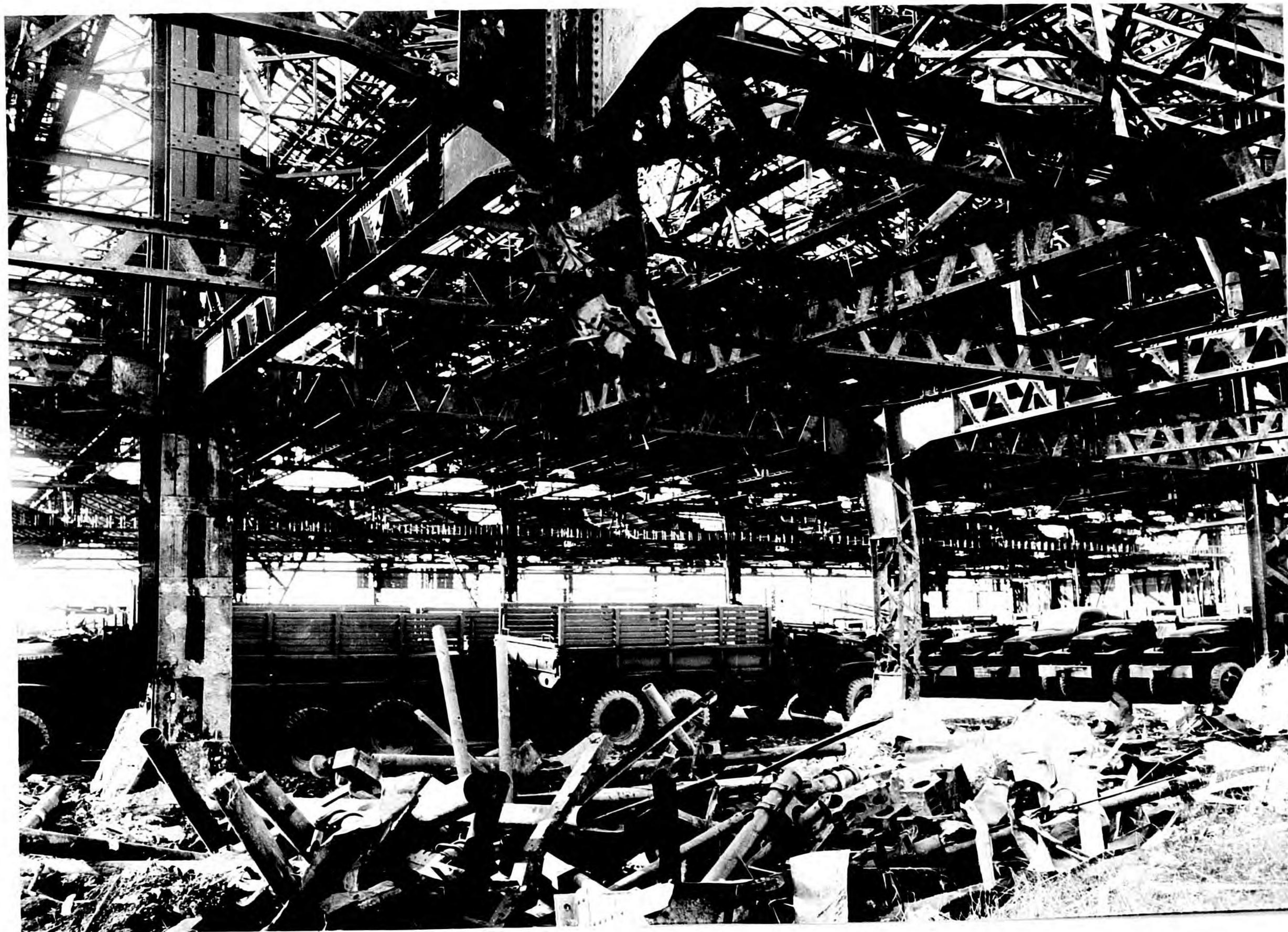
Photo 204. Large sections of this steel building stood without apparent distortion after columns were cut.
