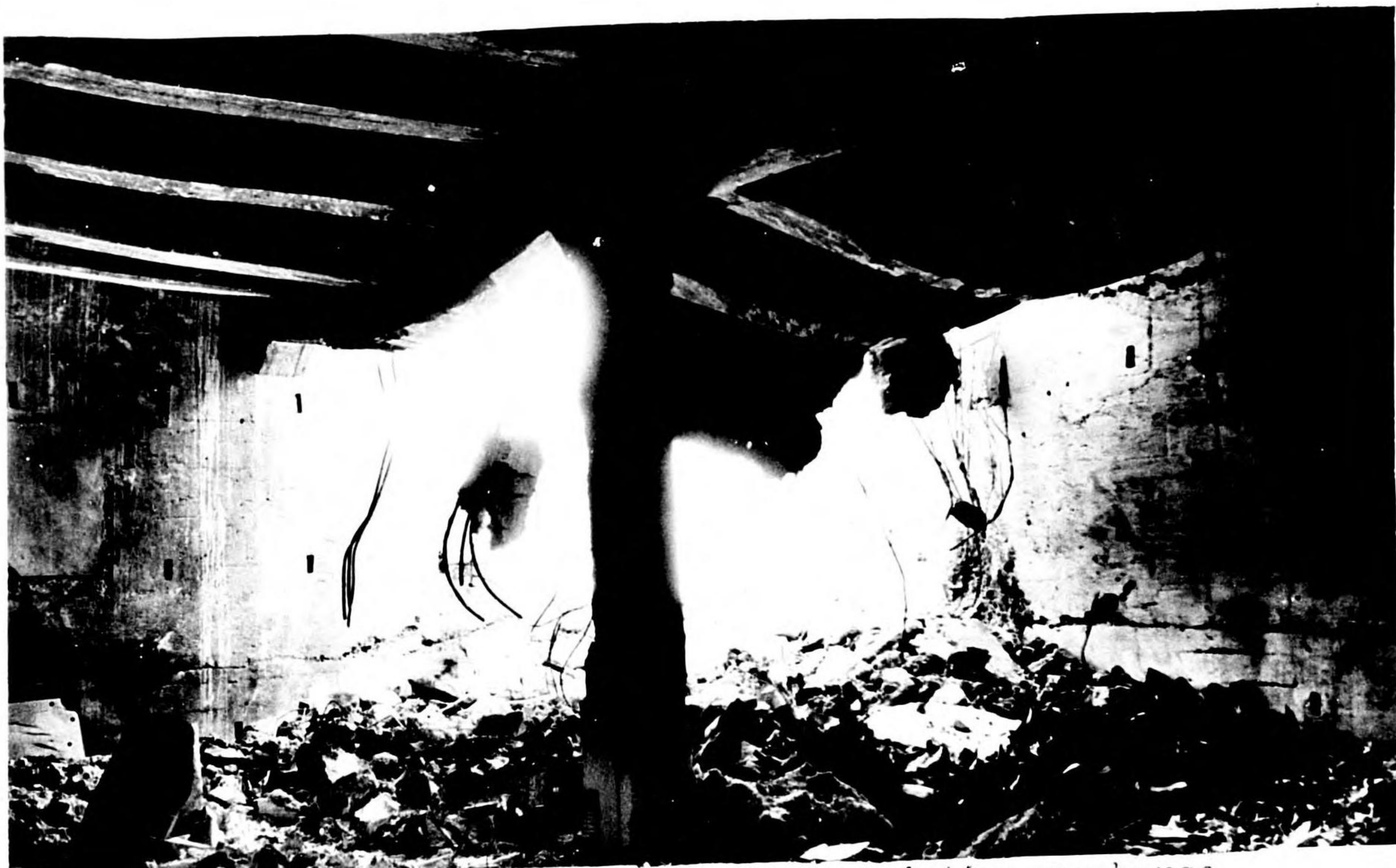
Photo 190. Hiroshima. Misasa Credit Association warehouse, reinforced-concrete building 5,800 feet from GZ. Second story of east section showing structural fire damage to roof, cracks in walls spalling of concrete on columns, and deep ashes on floor.
