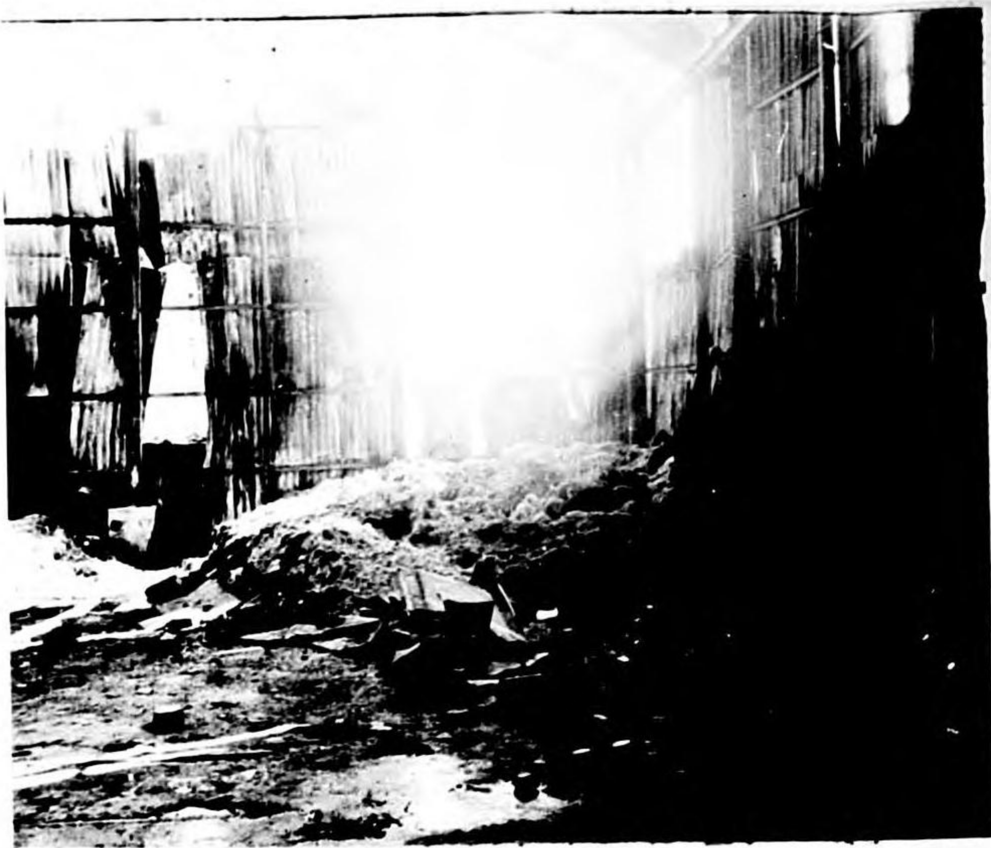
Photo 192. Nagasaki. Steel-frame building 6,400 feet from GZ which suffered heavy superficial and slight structural damage from blast. Combustible debris burned.
