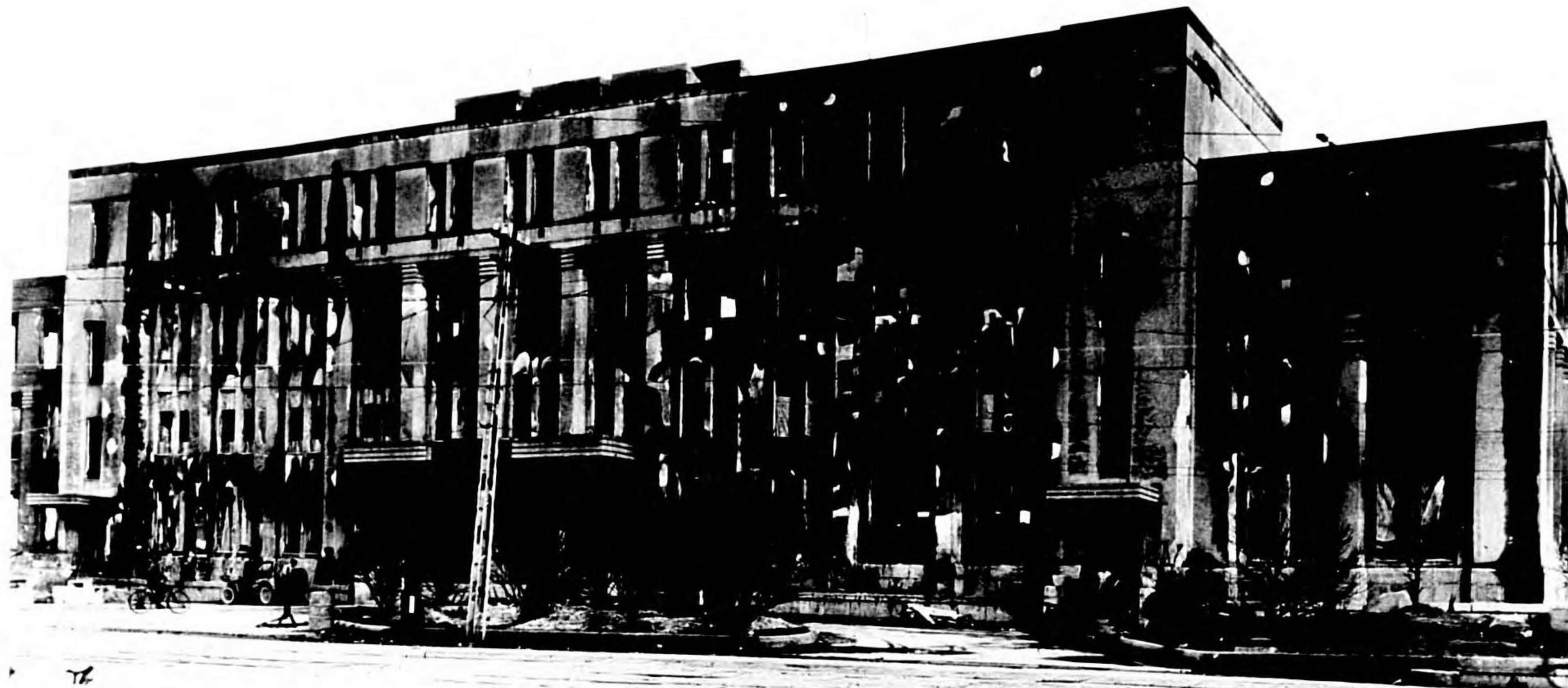
Photo 188. Hiroshima City Hall, 3,300 feet from GZ. West elevation of reinforced-concrete building--minor damage only: sash blown out, trim and finish consumed by fire. Few tile partitions blown out.
