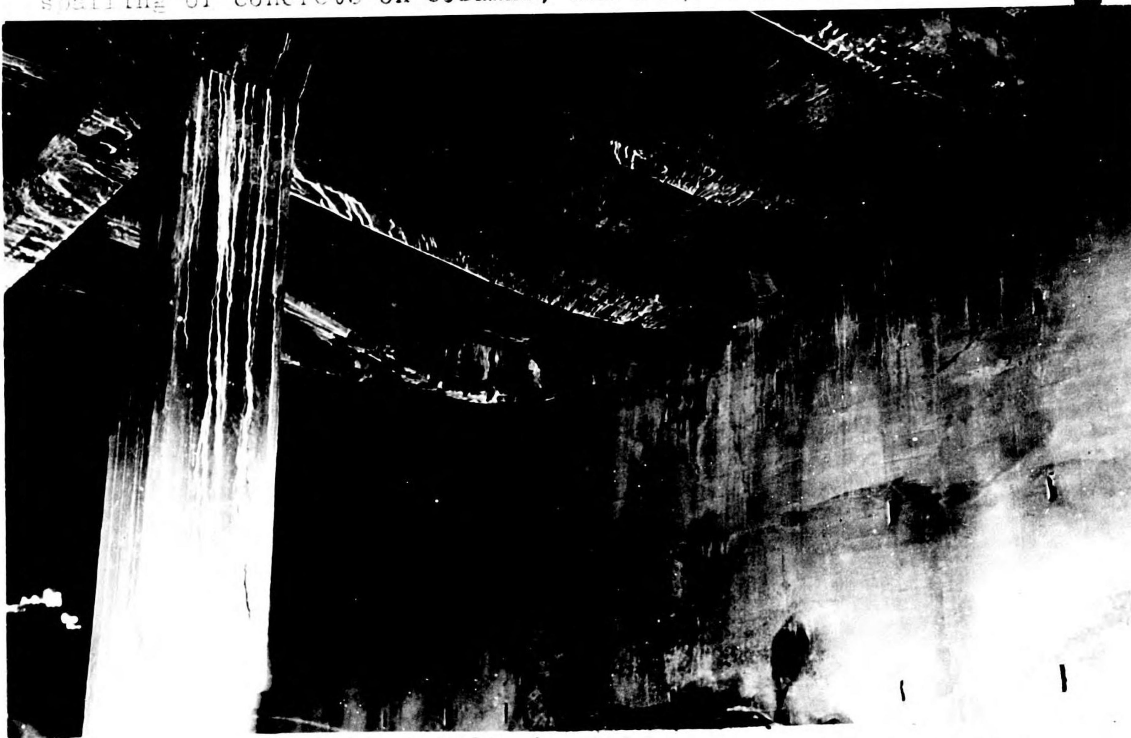
Photo 191. Same as Photo 190. View of first story showing structural damage to second floor by fire: spalling and disintegration of concrete.
