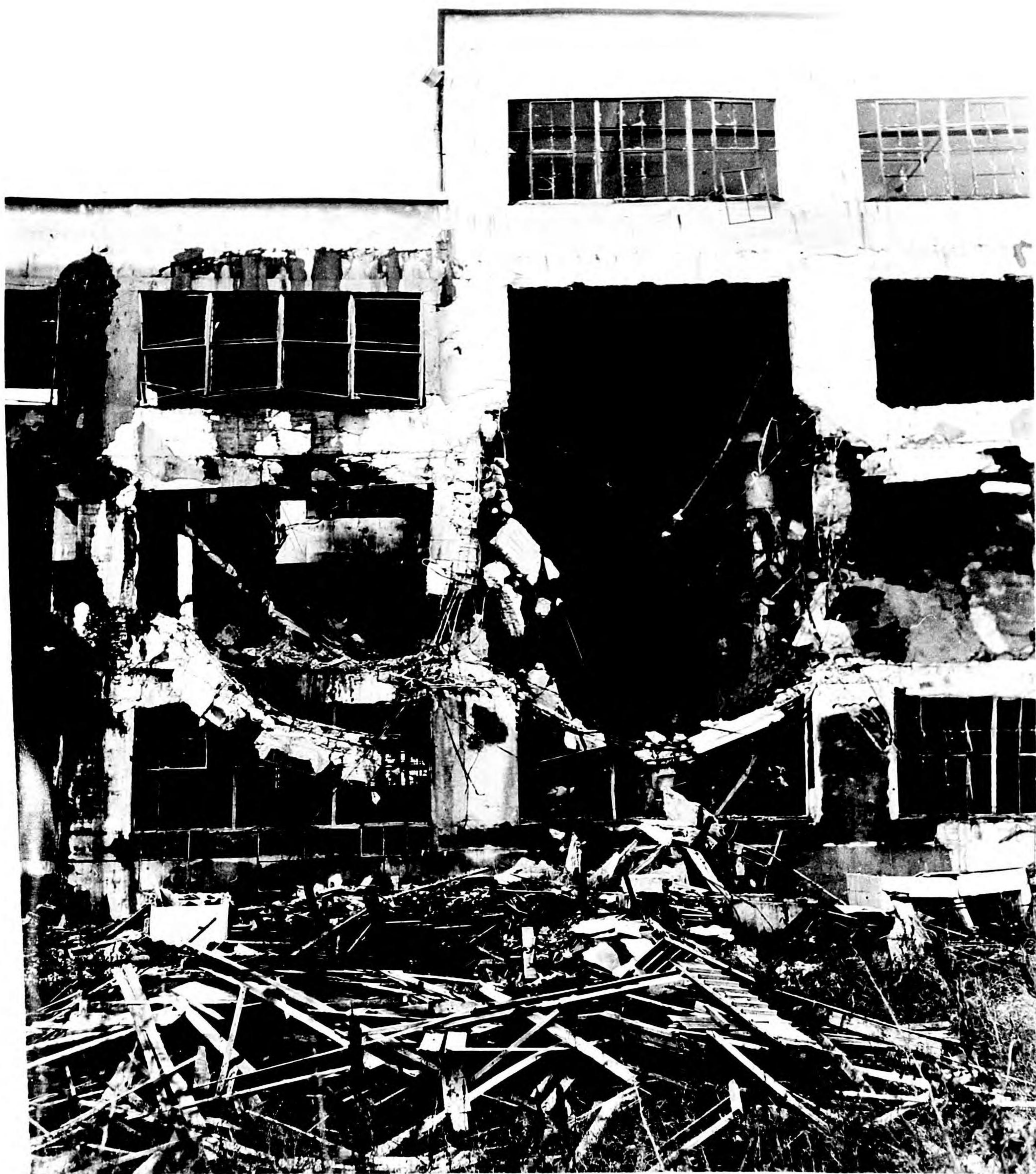
Photo 206. Another example at other end of building shown in Photo 205.
