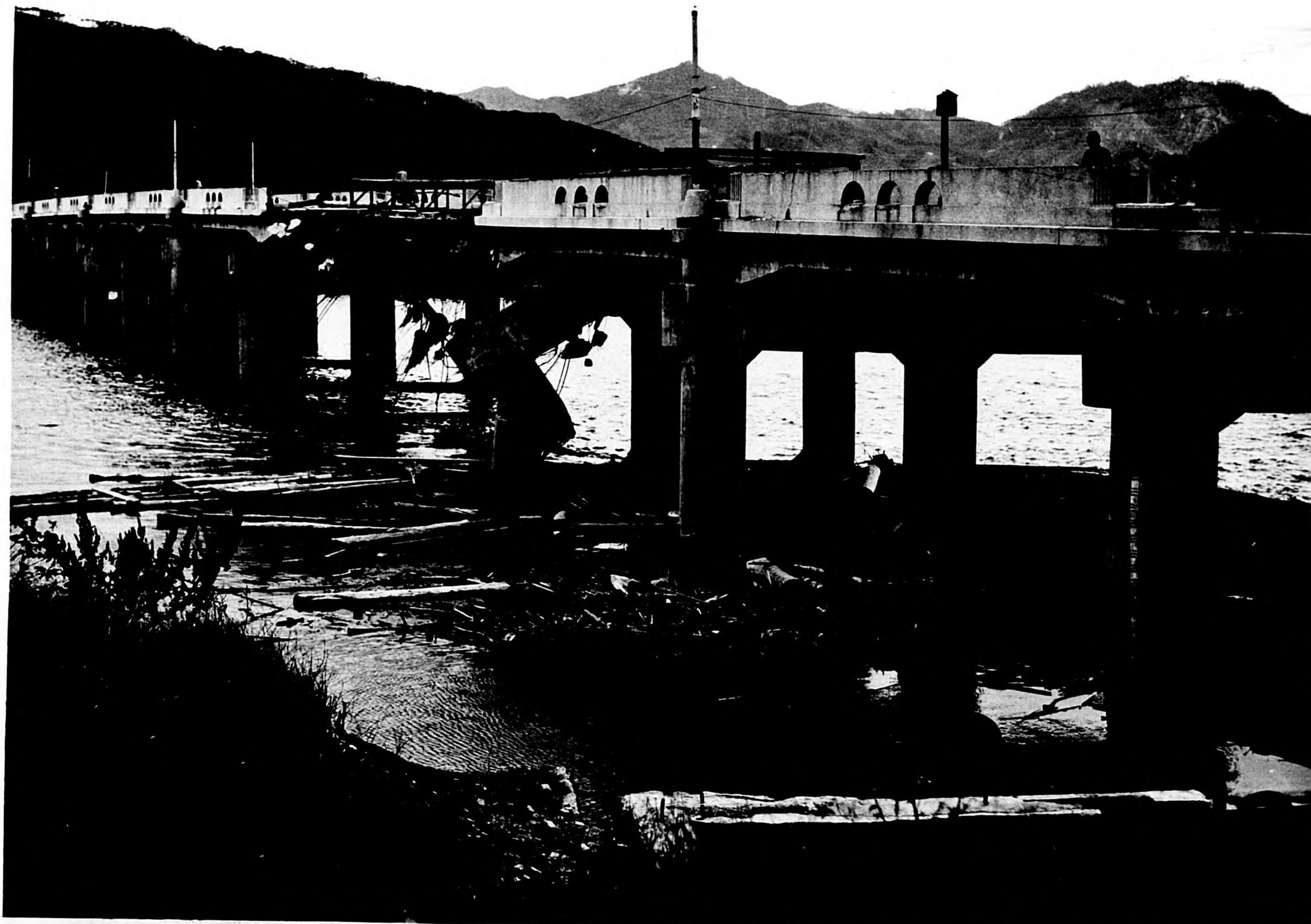
Photo 198. Reinforced-concrete bridge lost bent in flood. Adjacent bent was also severely damaged, but one-half of roadway remained in position and continued to carry unrestricted traffic.
