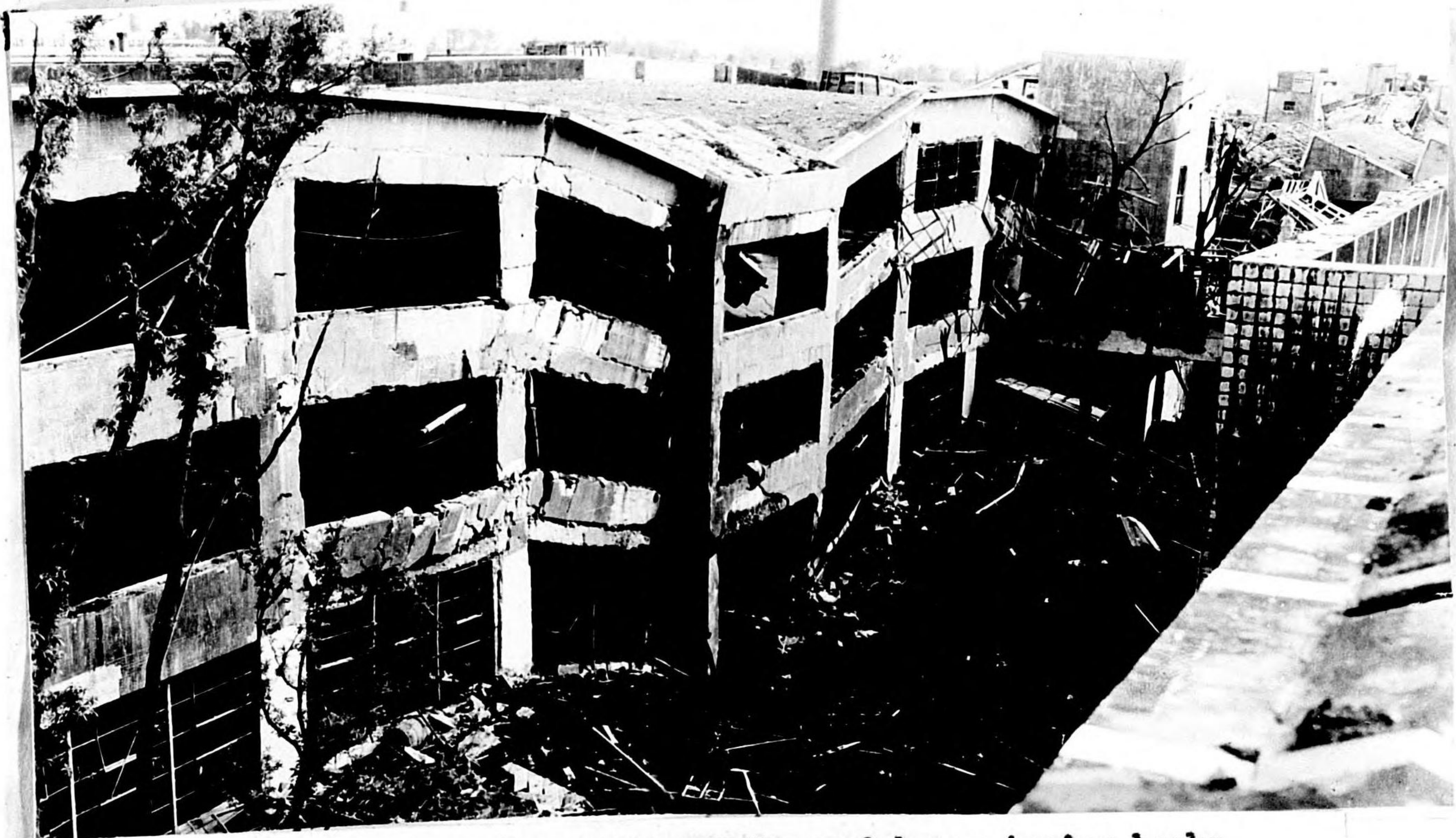
Photo 207. Bay and stairwell lowered by cratering bombs.
