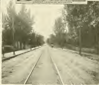
JEFFERSON ST. FROM S.W. CORNER
