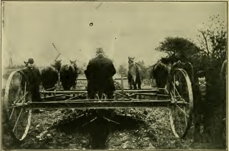
THE DITCHER IN OPERATION.
