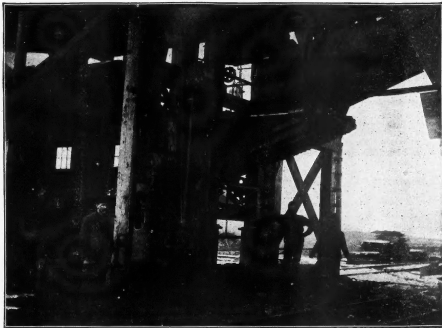
OTTUMWA COAL CONVEYOR.
