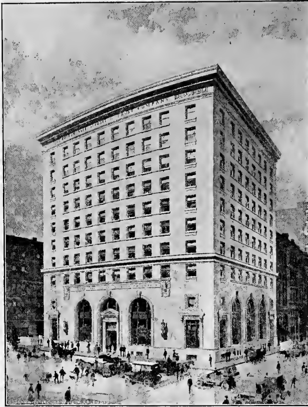
BOSTON SAFE DEPOSIT & TRUST CO. BUILDING DEVONSHIRE, ARCH AND FRANKLIN STREETS, BOSTON
