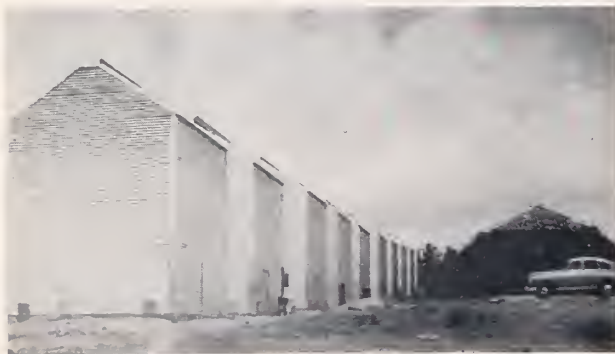
Typical flue-curing barns at Kurunegala, an important curing center. Made of corrugated iron sheeting, these barns are 16'x16'x20' and hold about 70,000 leaves.
