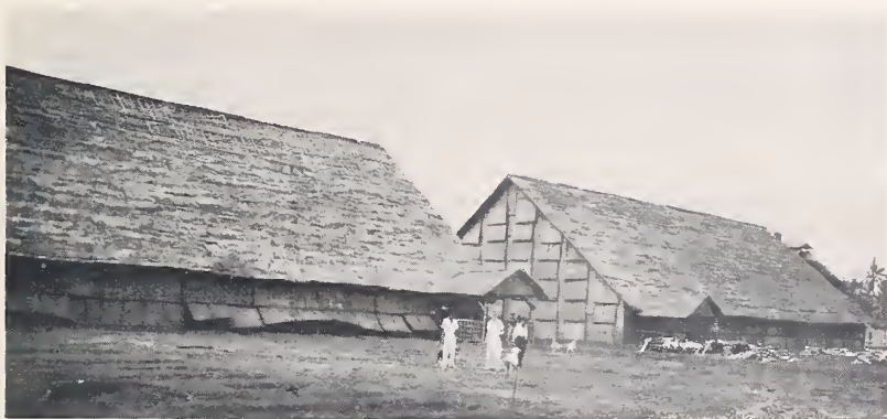
Left. Cigar leaf curing sheds in East Java made of palm-leaf matting supported by bamboo poles. Sections of matting on the sides and ends may be opened or closed for ventilation purposes. These sheds are 90 to 120 ft. long and 60 ft. wide.
