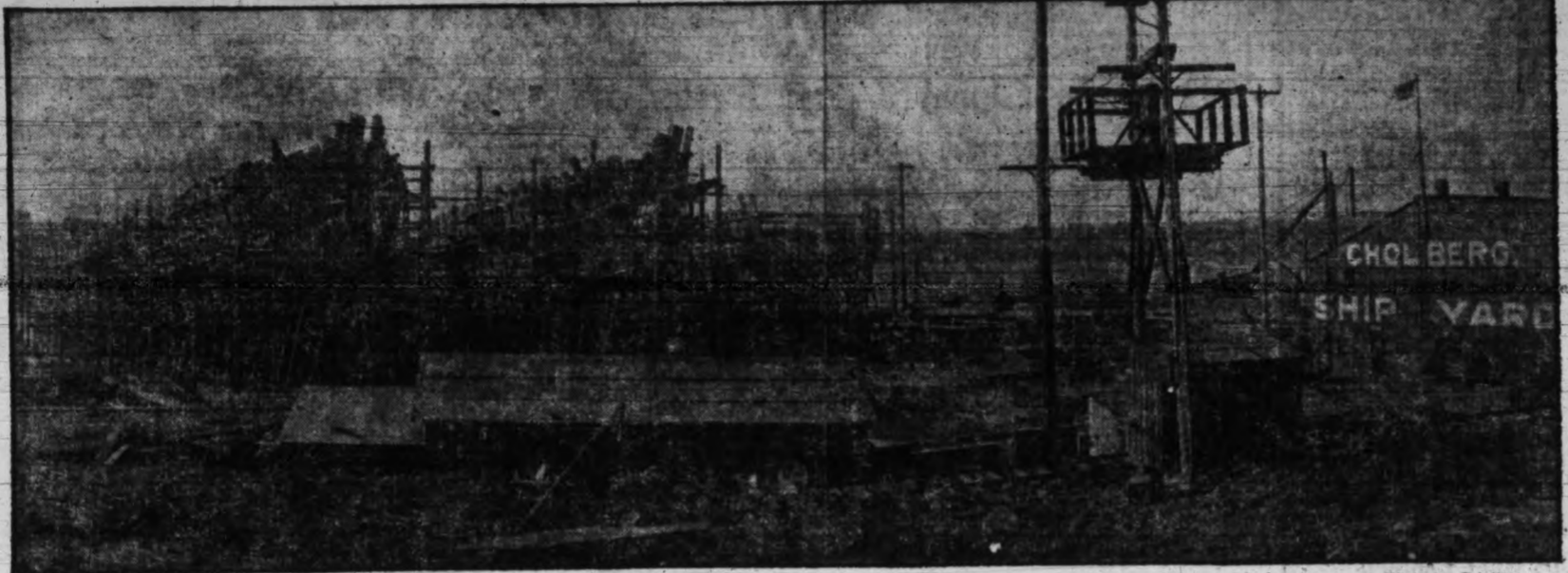
Showing three of nine four-masted 1,500-ton wooden schooners which the Cholberg Ship Company has contracted to build for Norwegian shipping interests. This three-way yard commenced operations six months ago when fresh ground was broken at Mud Bay on the south side of the old Songhees Reserve. Reading from left to right the vessels will be named Washington, Gunn and Vancouver. Planking is under way on the Washington and Gunn and it is predicted that the first of these ships will be ready for launching by the end of March.
