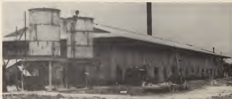
Figure 9. - The palm oil processing plant at San Alejo, Honduras.
