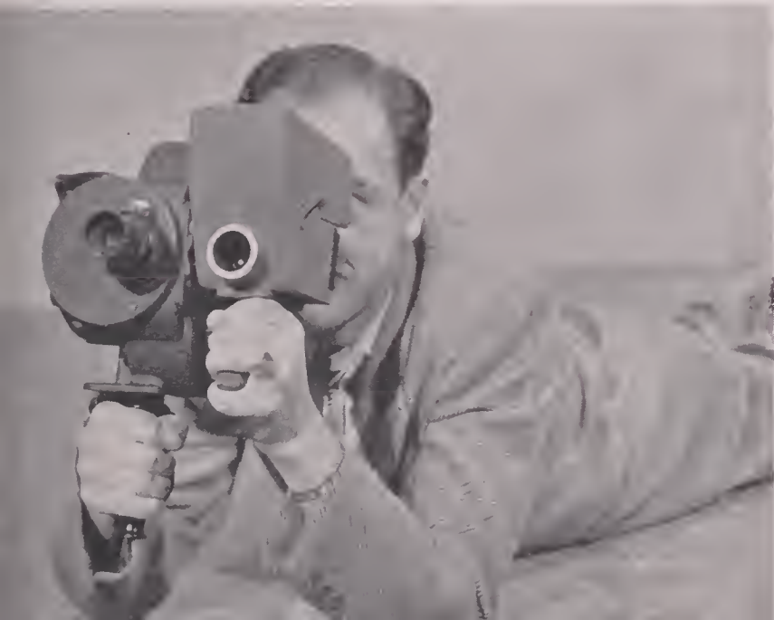
Bottom left, without tripod, "pistol-grips" on finder and camera provide means for shooting steady pictures in any position.
