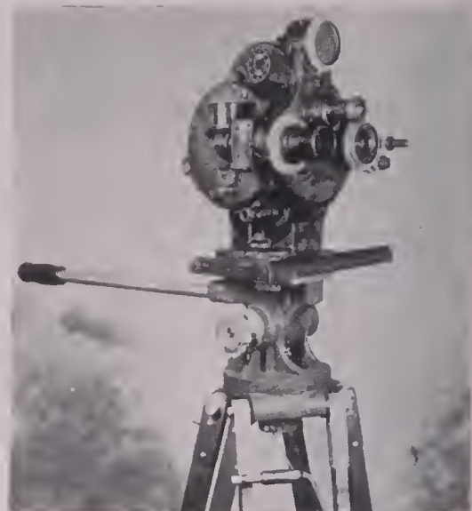
Eyemo turret showing side view of prismatic focusing magnifier.
