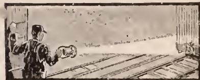
SHOVING TO A JOINT.
