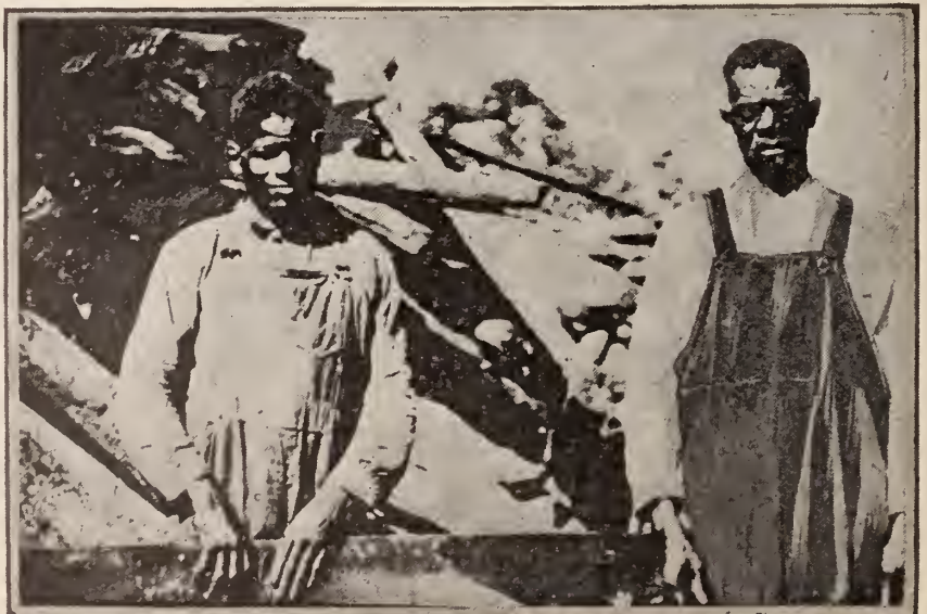
Leslie Green and R. T. Thompson, Maintenance Department, who sawed up hundreds of cross ties to keep the fires burning at the Water Pumping Station at Swan Creek, Md., during coal strike
