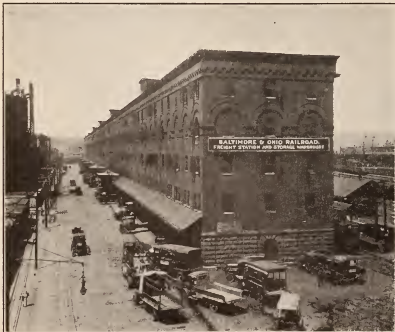
Smith Street Station and Warehouse, Cincinnati, Ohio
