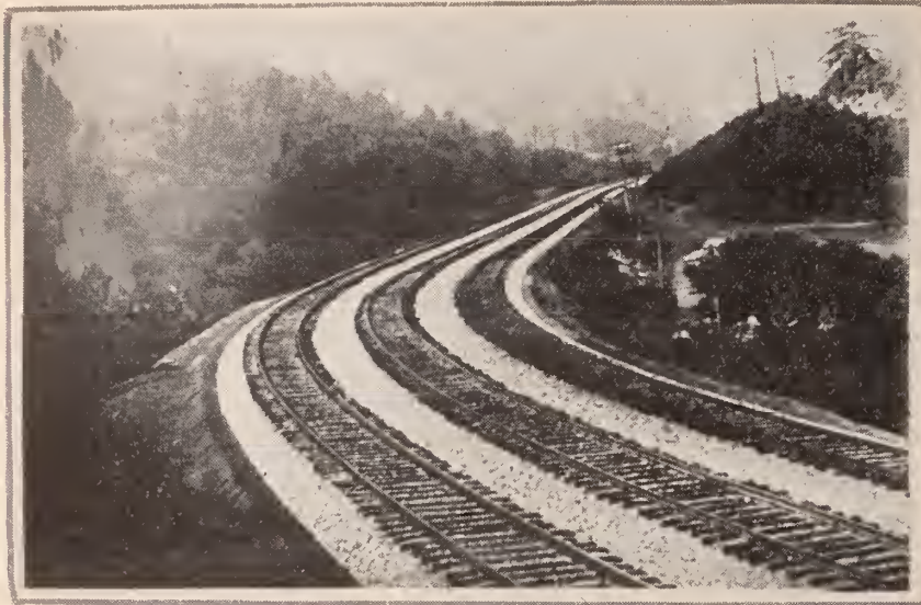
Standard Track, Baltimore and Ohio Railroad, Newburg Grade, Cumberland Division
