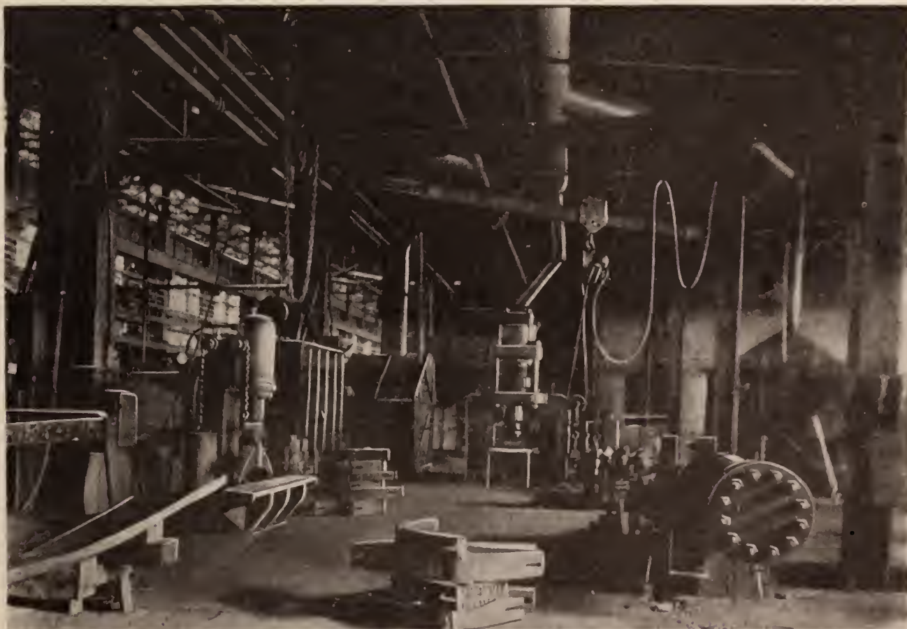
The orderly little Spring Plant at Glenwood
