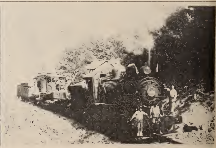
American ditcher No. 1, out on the line o'road
