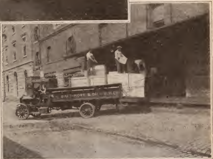
Delivering chute in operation, minimizing delay to teams; Baltimore, Md.
