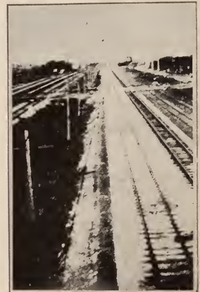
Standard Track, Baltimore and Ohio Railroad, west of Wheeling, W. Va.
