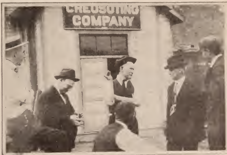
Superintendent Bade, Central Creosoting Co., telling Engineer Maintenance of Way S. A. Jordan about thorough penetration. The other interested listeners are, left to right: Plant Inspector Kittle; W. P. Abbott, former assistant division engineer, Cincinnati Terminals; Division Engineer J. H. Hewes, Jr., St. Louis Division; Signal Supervisor J. W. Kunker, St. Louis Division and Cincinnati Terminal
