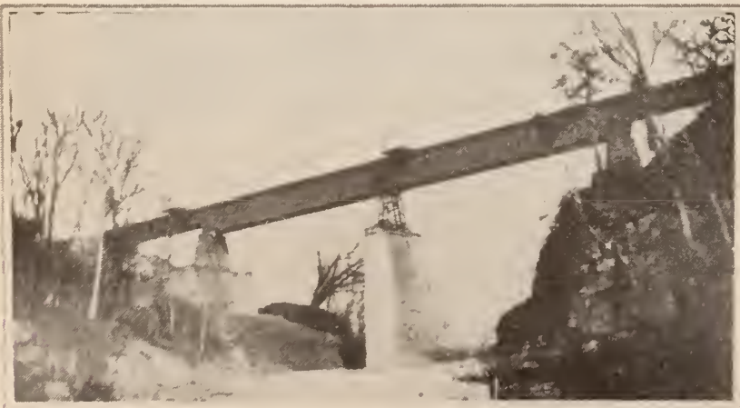
Bridge 67/65, over Rattlesnake Creek, Ohio Division
