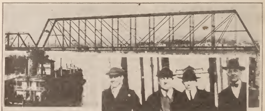
BRIDGE No. 935, LOOKING NORTH TOWARDS THE OHIO RIVER Insert: Wich, McCabe, Ramming, Shaeffer, all Engineering Department boys
