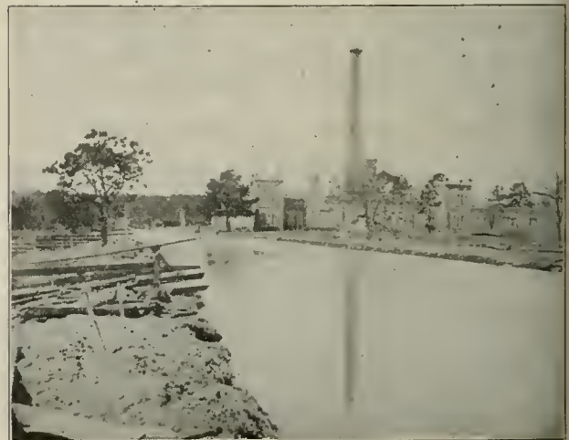
CHIMNEY OF OLD POWDER MILL, AUGUSTA, GA.
